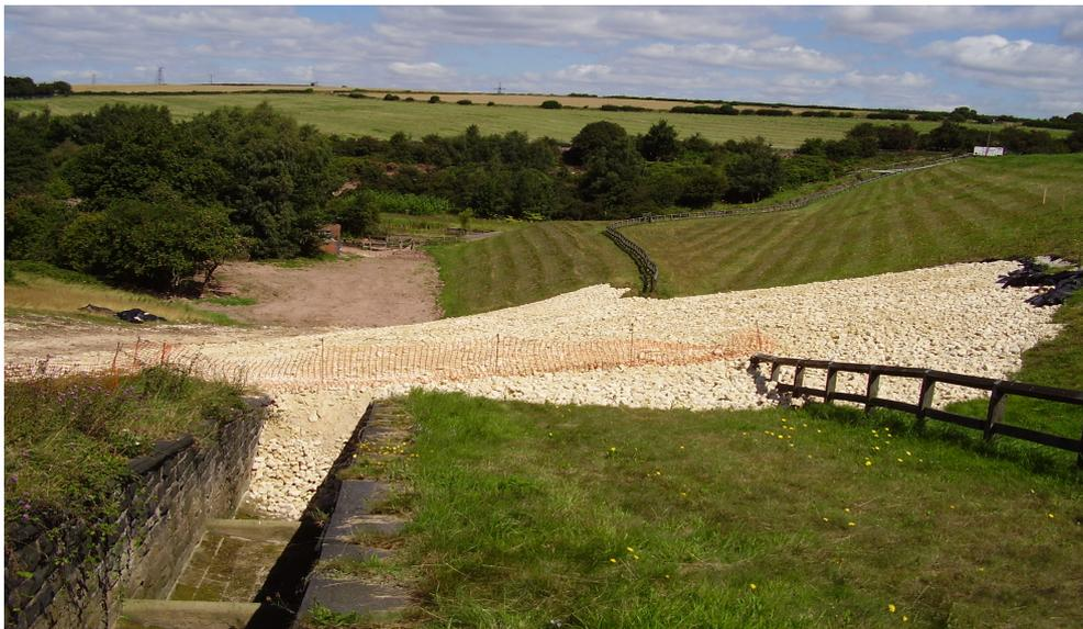
Figure 6 - Repaired scour hole after incident
