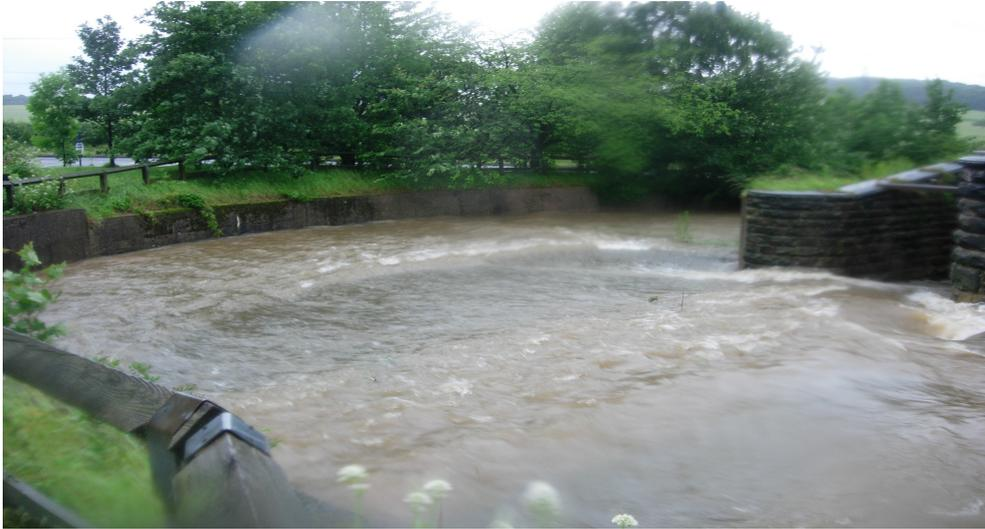
Figure 2 - Flow down 1943 spillway and original south spillway during the incident. Original south spillway is on extreme right of photograph.
