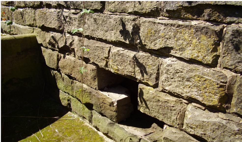
Figure 5 - Local hydrodynamic stone removal. Note also general condition of wall.
