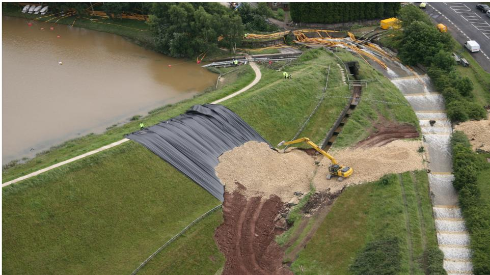
Figure 1 - Works in progress filling scour hole
