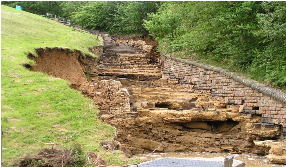
Figure 7 - Damaged spillway at Boltby in 2005
