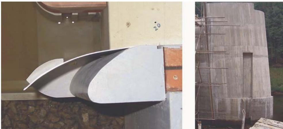
Figure 6. The stream-leading plate set on top of the lower part of the side pier and its realisation by a concrete body with a groove of the cofferdam
