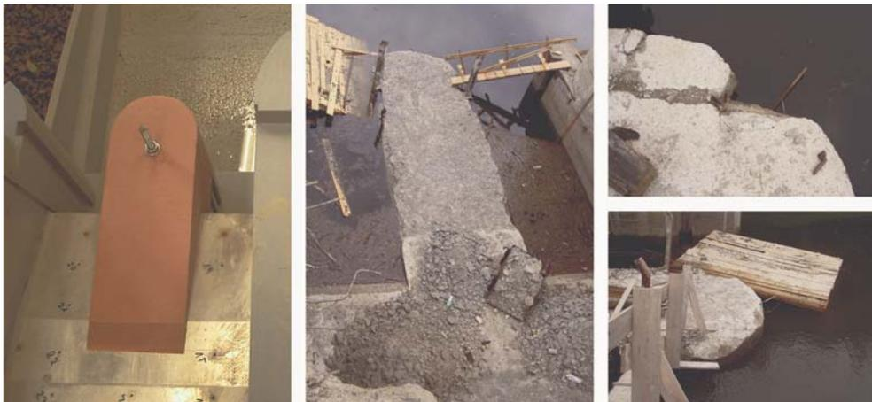
Figure 3. Recommended and applied modification of separating piers
