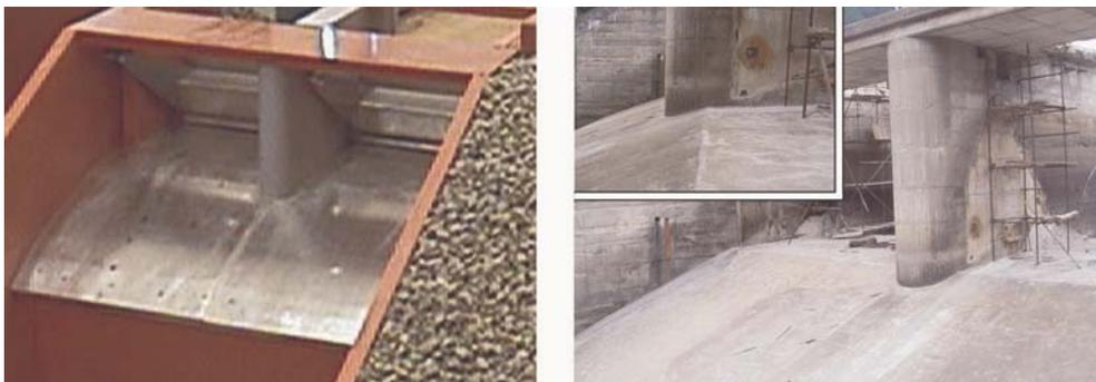
Figure 4. Modelled and realised shape of the spillway surface at the end of central pier
