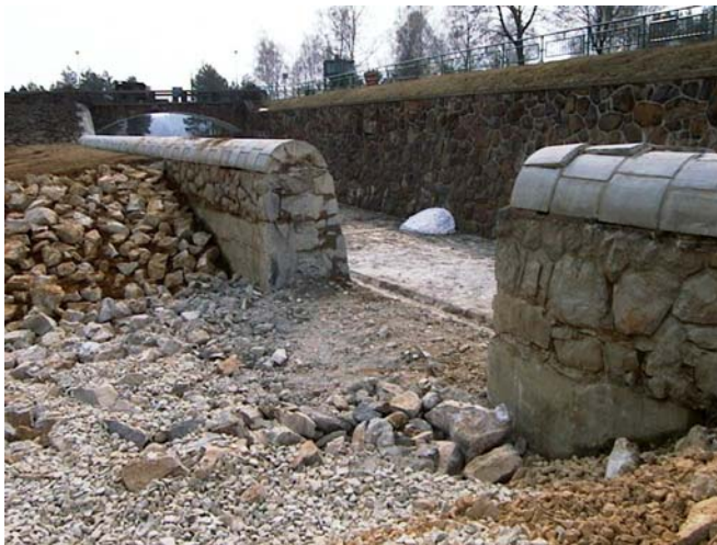
Figure 4: Emergency spillway - partial removal of spillway wall
