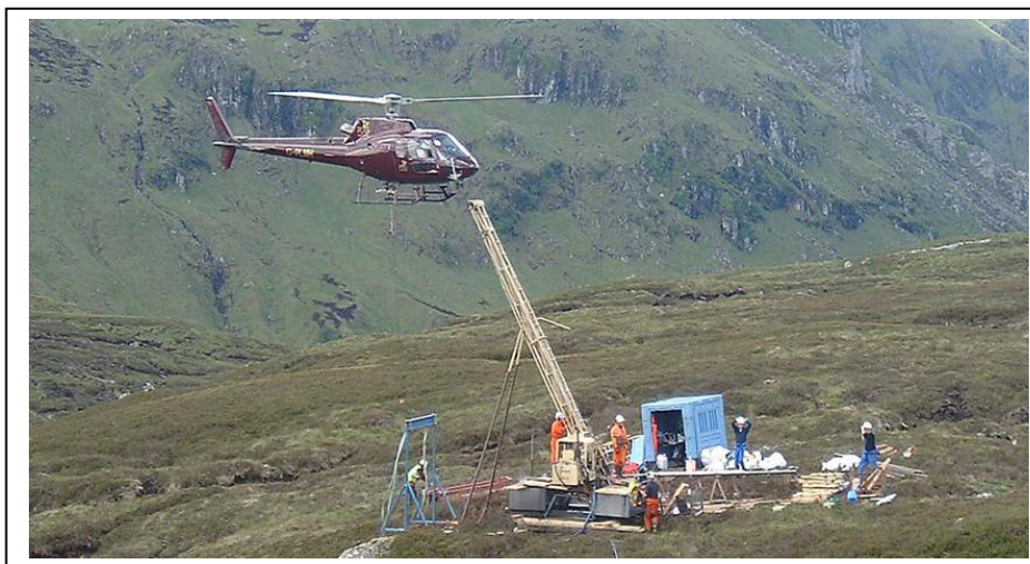
Figure 3. Dam Site Investigation
