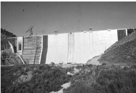
Figures 2 & 3: Pracana 65 m high buttress dam in Portugal, affected by AAR, was waterproofed with an exposed PVC liner in 1992. In 2003 (at right), the owner reports “the concrete dam waterproofing may be assumed to contribute for the reduction of the swelling process”.
