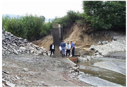
Figure 4: Melin – dam breach with remaining service shaft of the bottom outlet
