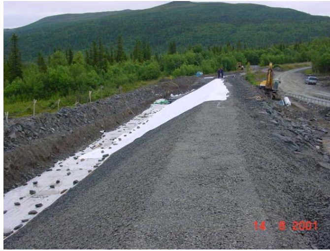
Figure 8. Placing of geotextile on the compacted coarse filter bedding. The textile is temporarily held in place by rocks.
