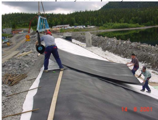
Figure 8. Placing of geotextile on the compacted coarse filter bedding. The textile is temporarily held in place by rocks.
