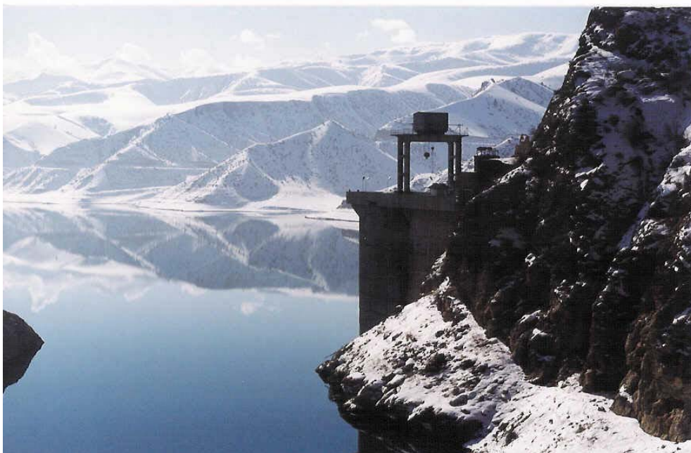
Figure 5. Papan dam – Reservoir and Intake Tower
