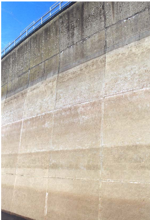
Figure 2: photo of existing shotcrete lining
