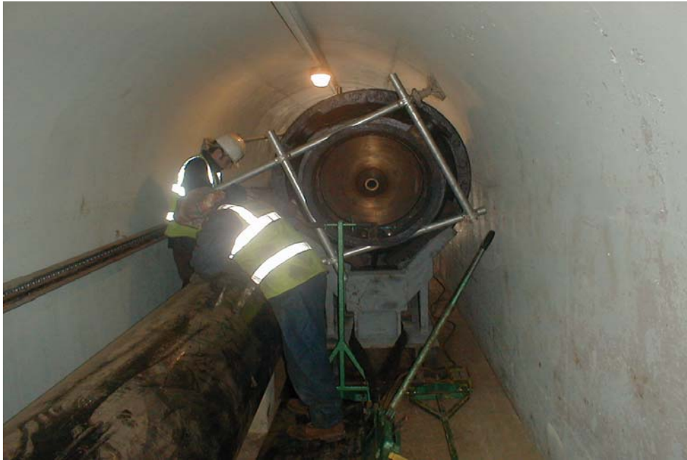
Plate 5: Transporting the Larner Johnson Valve
