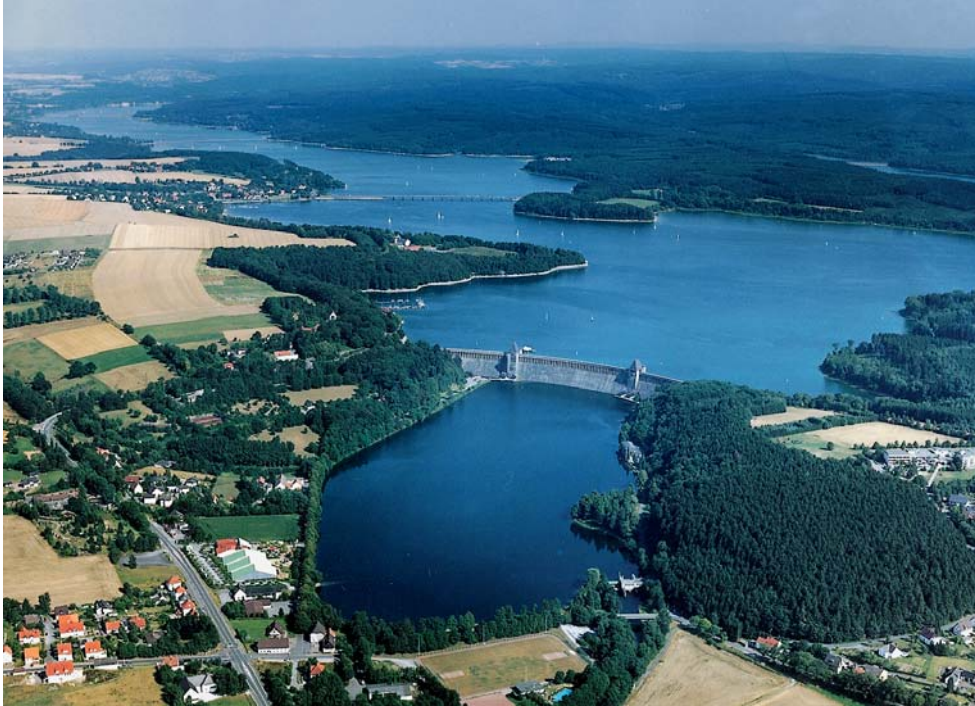
Figure 1. Aerial View of the Moehne Reservoir
