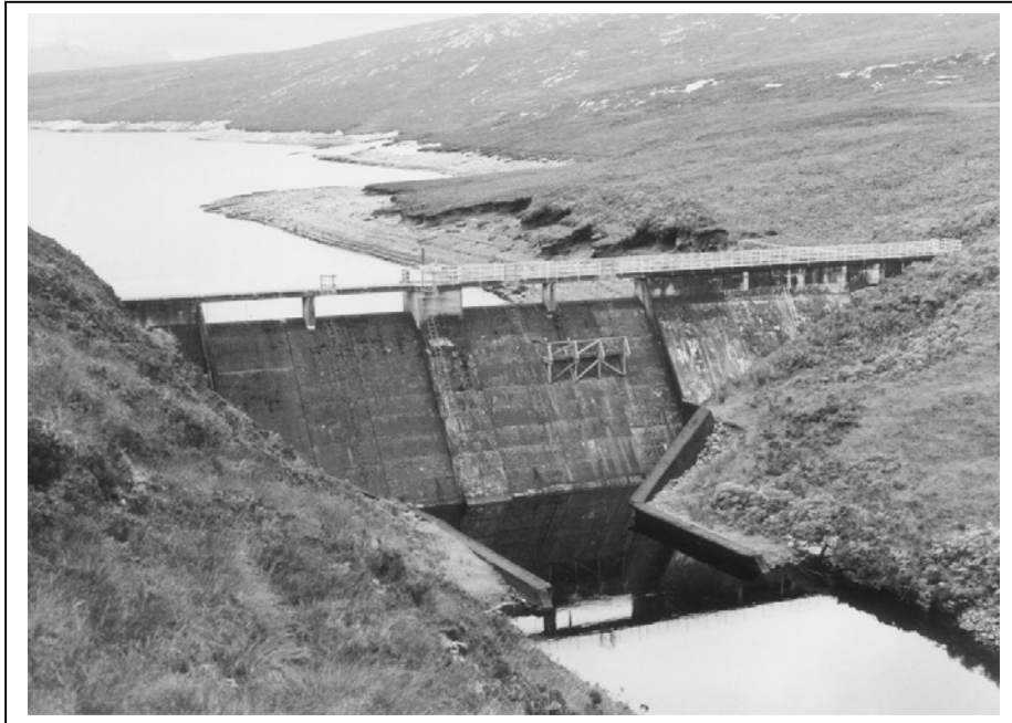
Figure 1: General View of Loch Dubh Dam
