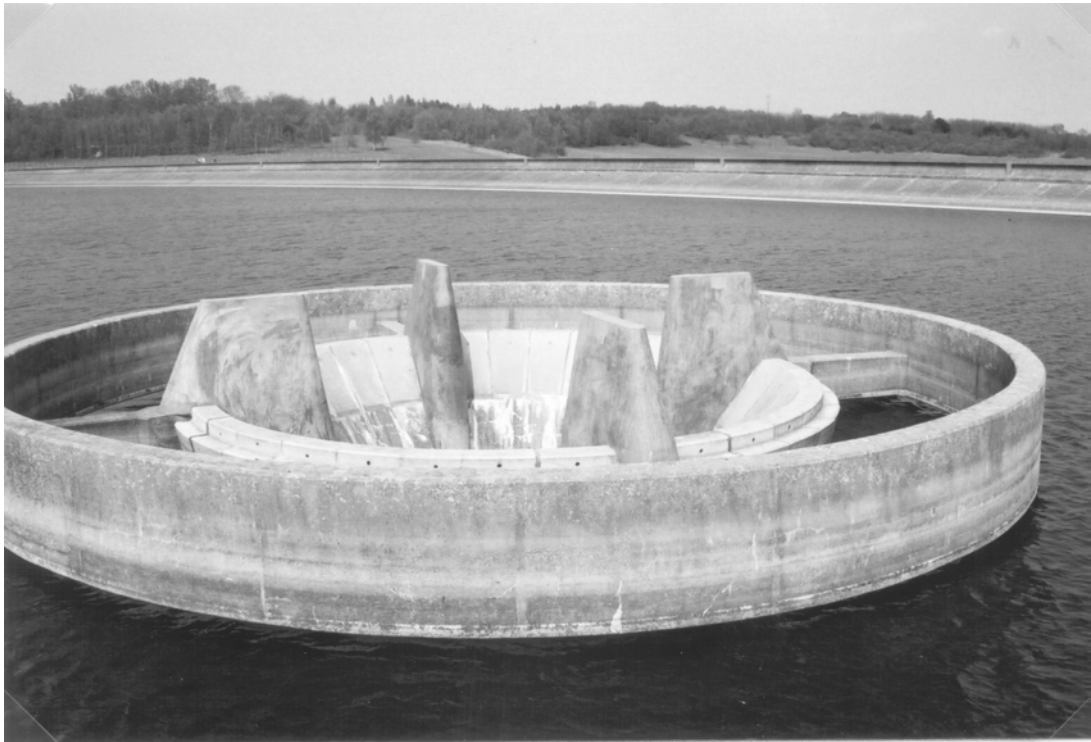
Figure 4 - Completed spillway crest
