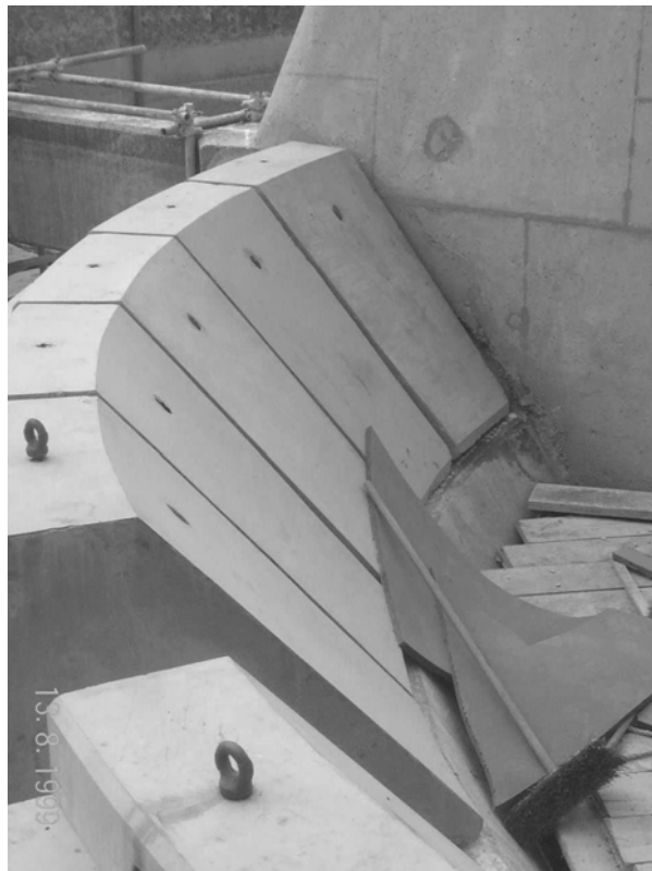
Figure 3 - New blocks in place
