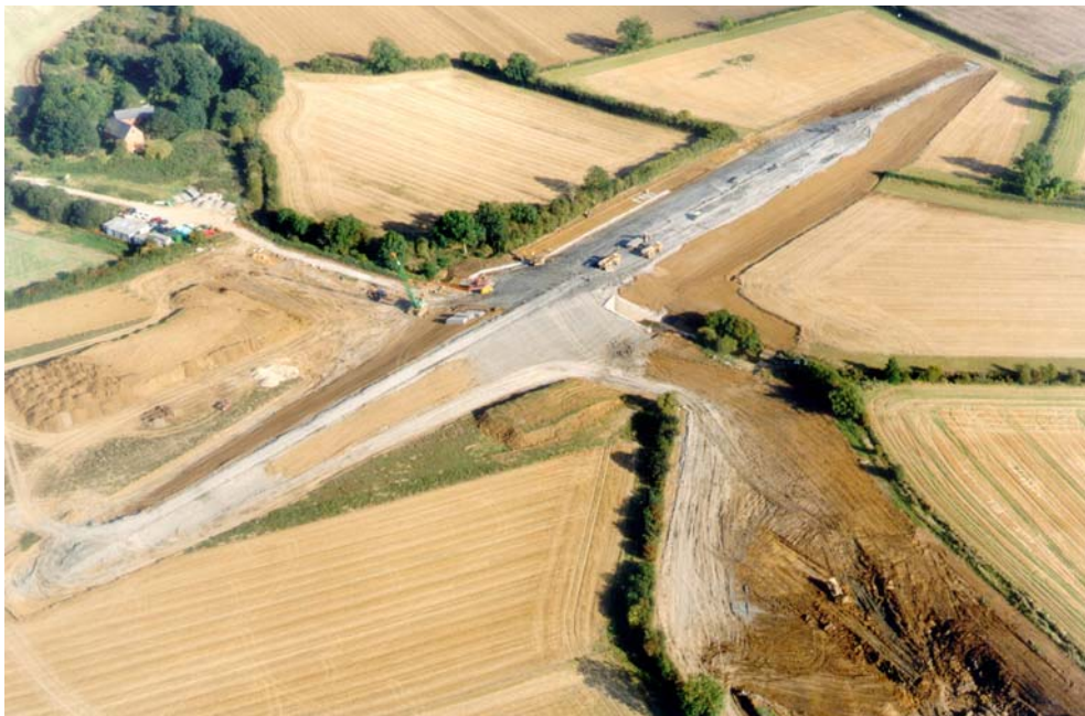
Figure 1: Weedon Dam under construction. The borrow pit is at the lower right. Note retained tree and hedge lines screening the embankment.
