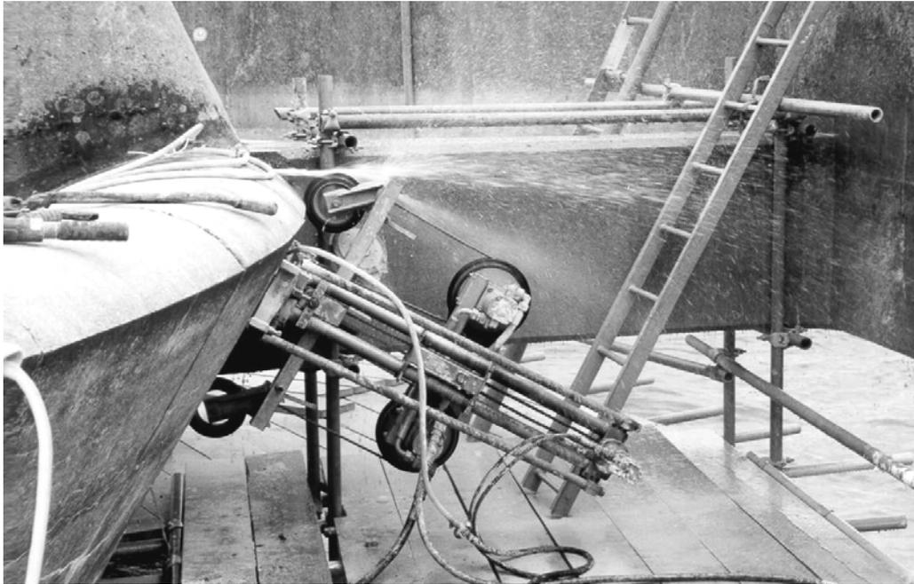
Figure 2 - Saw cutting between the existing blocks
