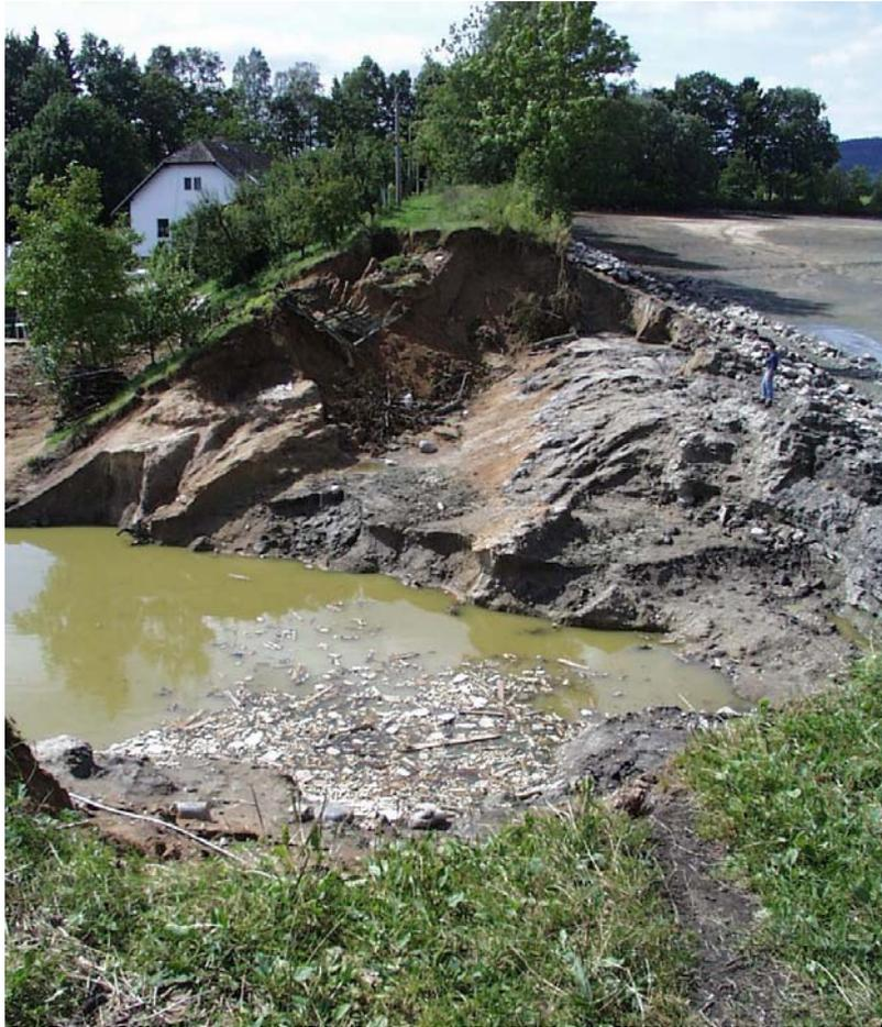
Figure 5: Dam Metelsky - the cross section at the right breach
