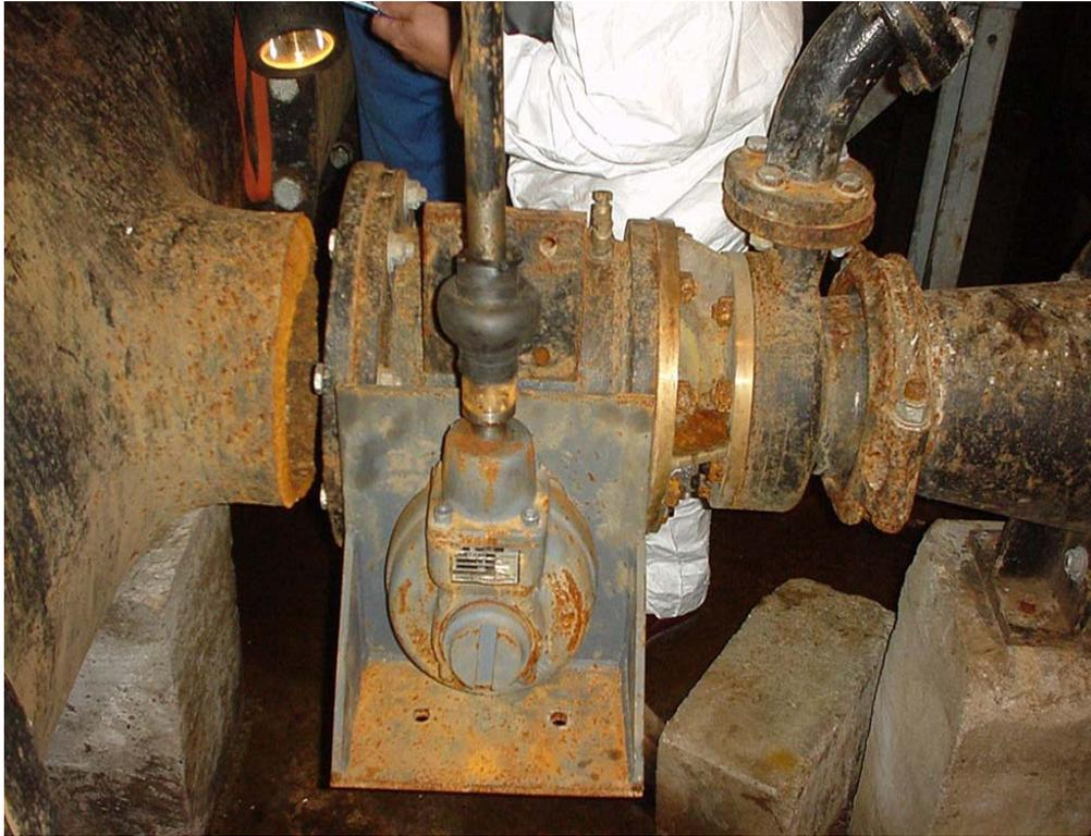
Plate 2: Fractured compensation pipework
