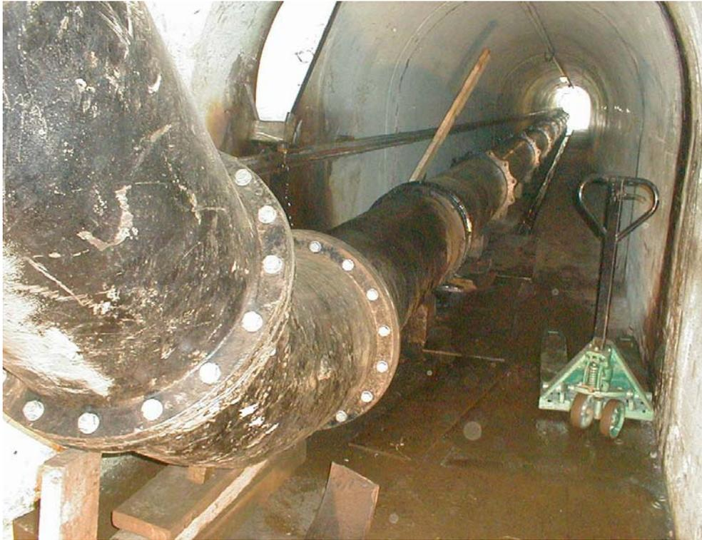
Plate 4: Draw-off main within the draw-off tunnel
