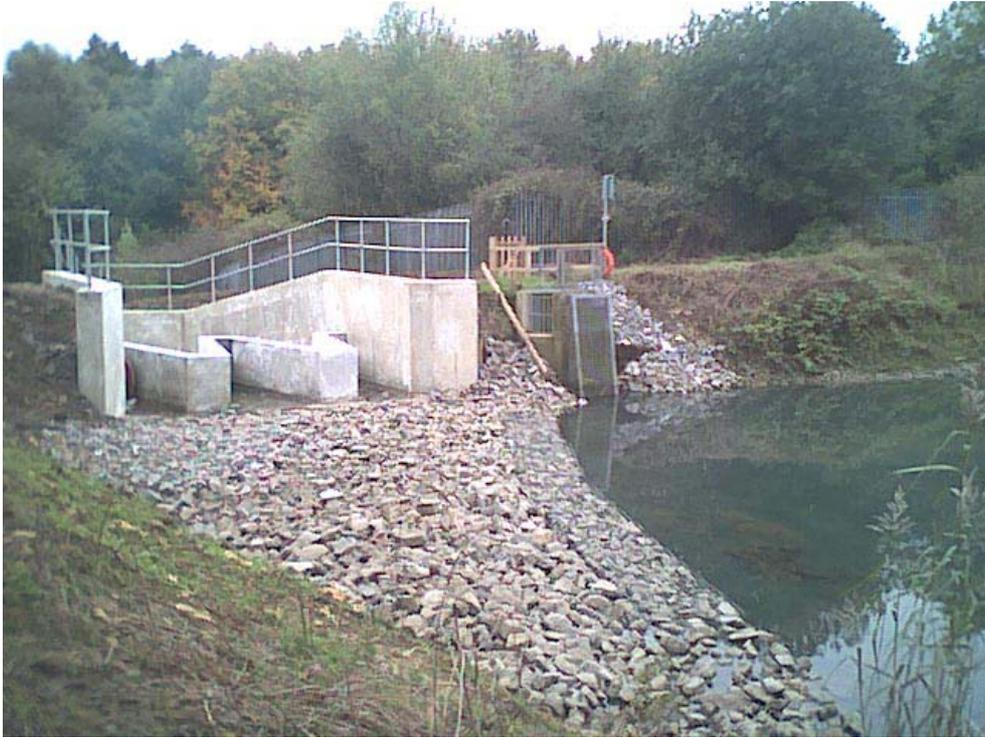
Figure 2. New Labyrinth Spillway at Weldon Lagoon
