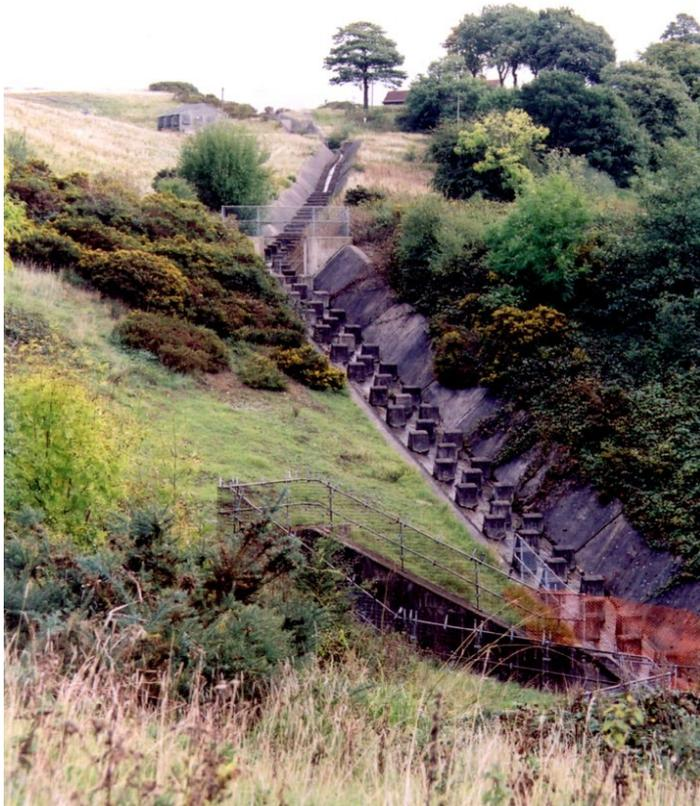
Plate 2: Eastern cascade channel on the left mitre of the embankment
