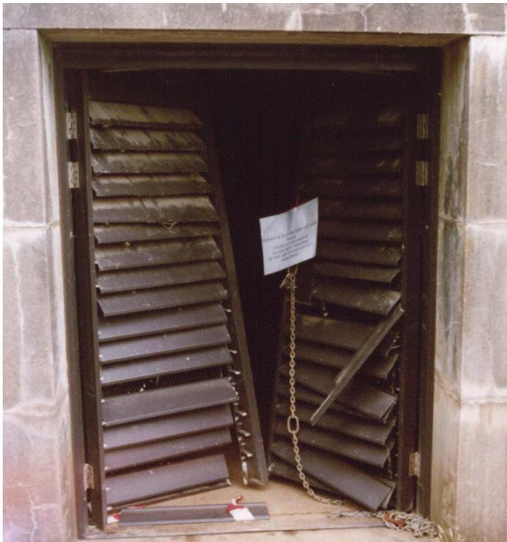
Plate 3: Damaged draw-off tunnel doors
