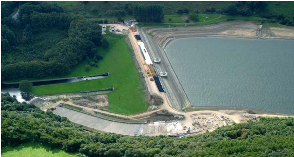
There are considerable benefits from being able to undertake iterative hydrology, hydraulic calculations and model testing at the same time. Changes to any one component can affect the others. For example, removal of spillway restrictions at Fewston and Swinsty changed the hydraulic characteristics, reduced the flood attenuation, and increased the required freeboard at Lindley Wood.
