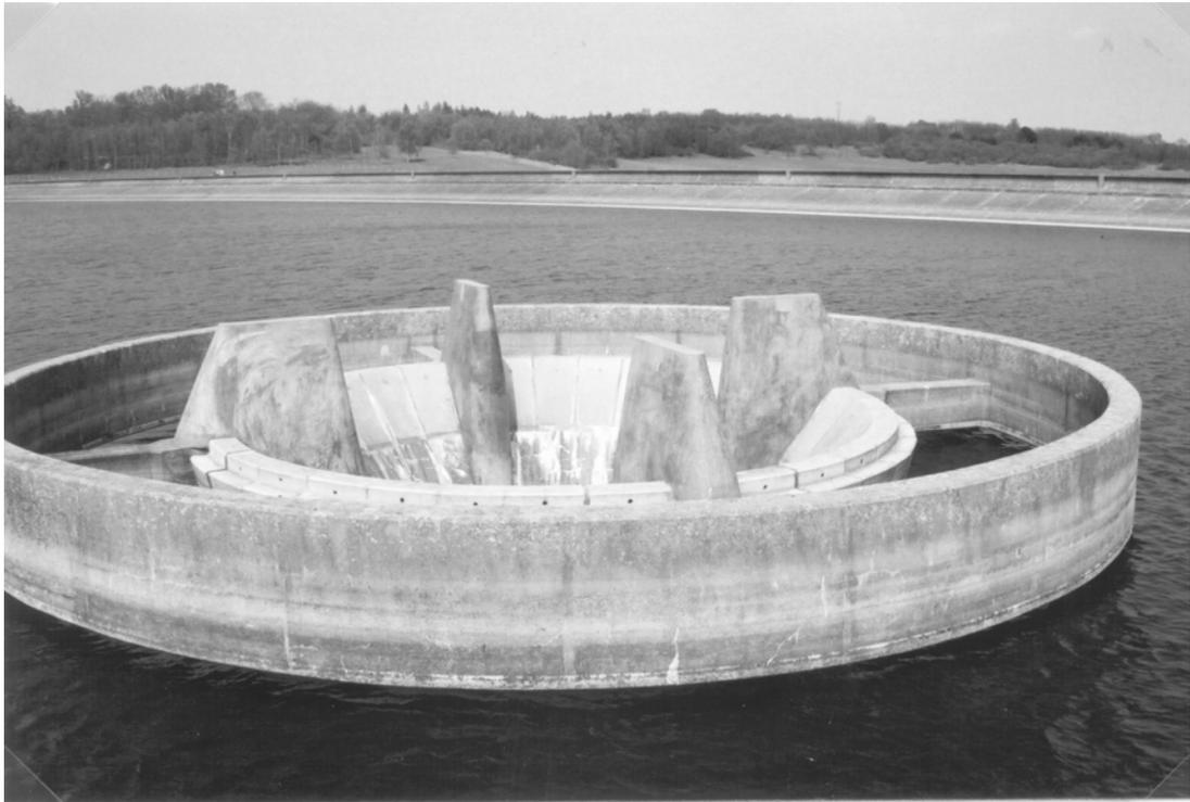
Figure 4 - Completed spillway crest
