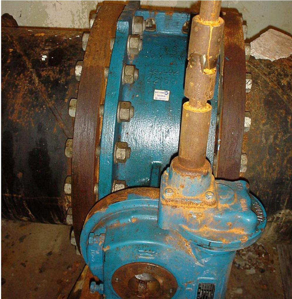
Plate 6: Failed butterfly valve in position and failed gearbox component
