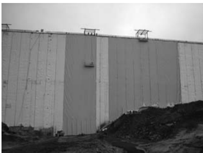
Figures 4 & 5: Beli Iskar 49.7 m high masonry dam, Bulgaria 2002. The exposed PVC geocomposite is installed on an anti-puncture geotextile. The dam is at 1878 m of altitude, ice thickness up to 0.60 m.
