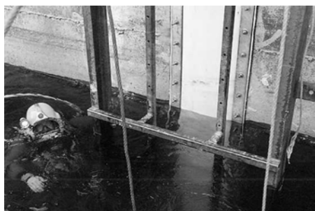
Figures 10 & 11: On the left, the external waterstops on the contraction joints of Porce II 118 m high RCC dam (Colombia 2000). The same external waterstops were installed in 1998 on Platanovryssi 95 m high RCC dam in Greece. In 2002, the external waterstop was used again at Platanovryssi, to repair a new crack that formed during first impoundment. Installation was performed underwater (on right).
