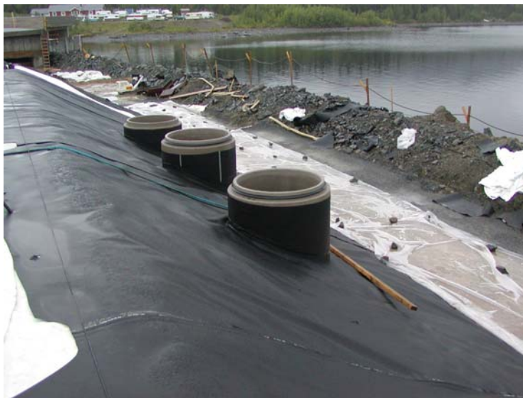
Figure 11. Protected connections through the membrane for instrumentation in the downstream filter.
