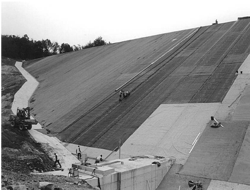
Figure 2: Work in progress at La Galaube
