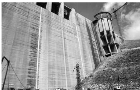
Figures 10 & 11: On the left, the external waterstops on the contraction joints of Porce II 118 m high RCC dam (Colombia 2000). The same external waterstops were installed in 1998 on Platanovryssi 95 m high RCC dam in Greece. In 2002, the external waterstop was used again at Platanovryssi, to repair a new crack that formed during first impoundment. Installation was performed underwater (on right).
