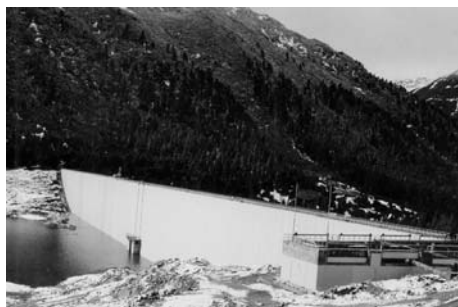
Figures 4 & 5: Beli Iskar 49.7 m high masonry dam, Bulgaria 2002. The exposed PVC geocomposite is installed on an anti-puncture geotextile. The dam is at 1878 m of altitude, ice thickness up to 0.60 m.
