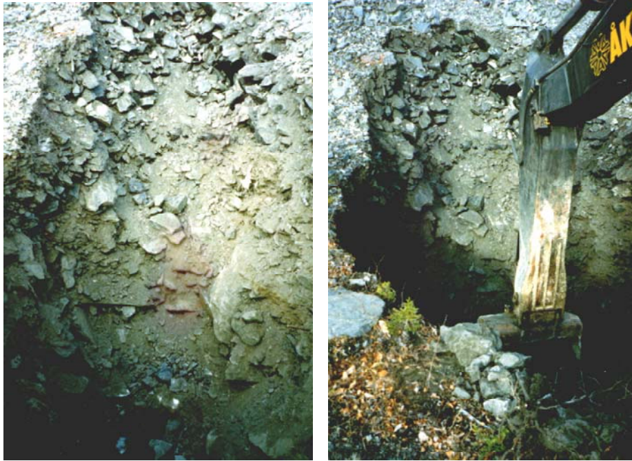
Figure 3. Test pits in the downstream toe of the original supporting fill
