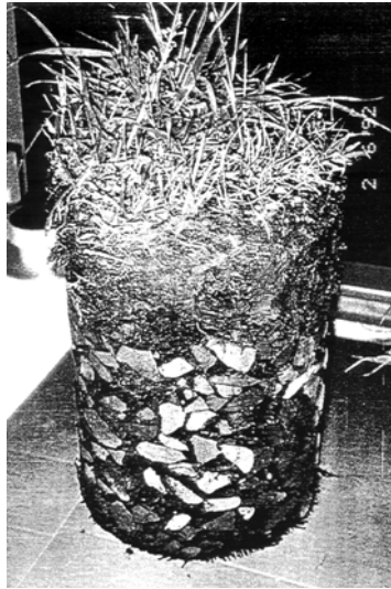
Figure 1: Drilling core extracted from a revetment of Open Stone Asphalt at the project Tielrode (B) with a layer of humus for planting vegetation (Source: ELSKENS 1995)
