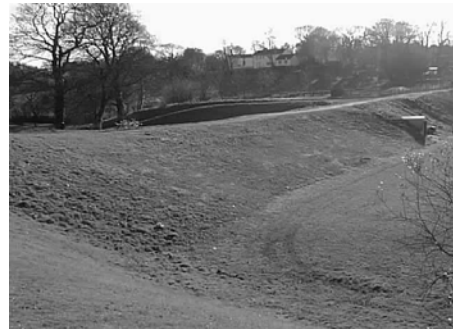
Fig 10: Downstream slope after topsoil/seedling
