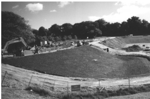
Fig 9: OSA erosion protection as installed
