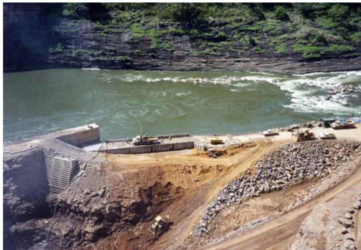
Capanda Powerhouse Cofferdam
