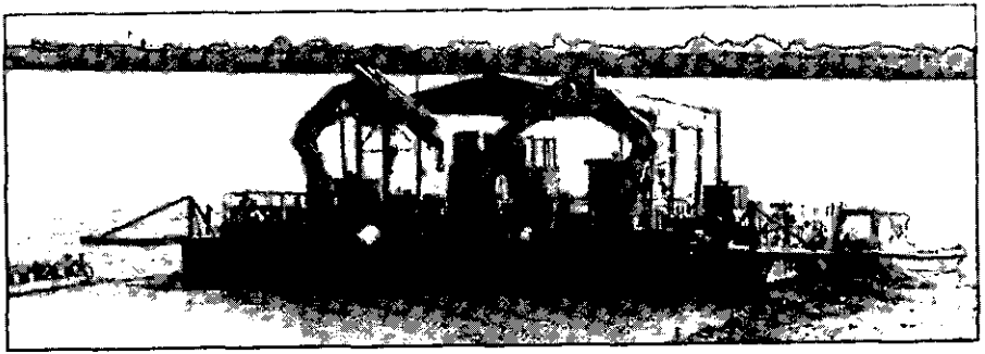
Fig. 6. Pontoon at foot of Slipway
