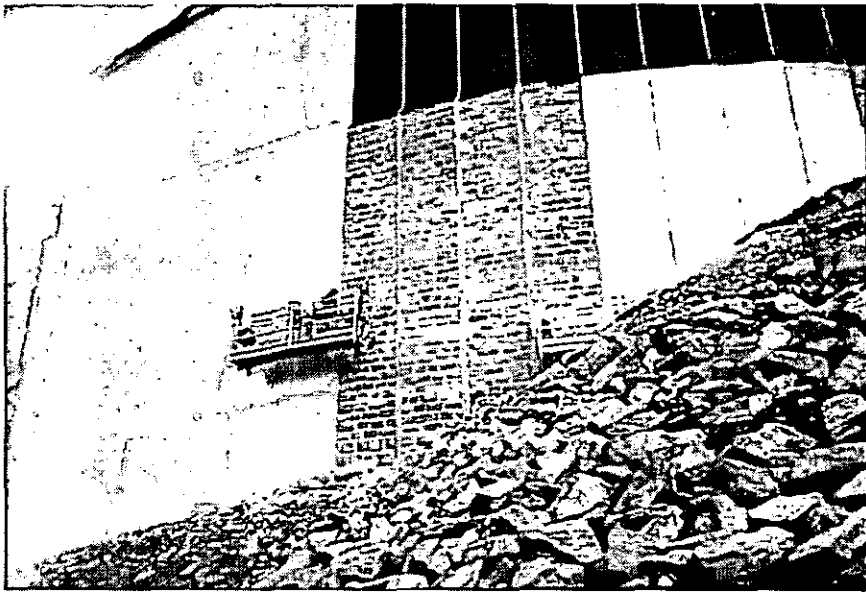
Figure 4.8 Illsee dam, geomembrane on the upstream face.
