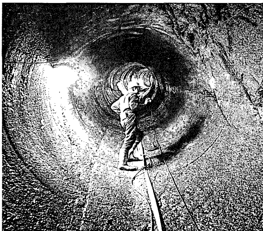
Figure 3.3 Ennepe dam, drainage gallery.
