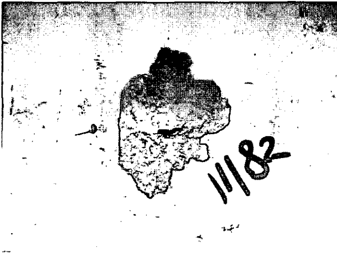
Figure 4.5 Kambura dam, concrete popout.
