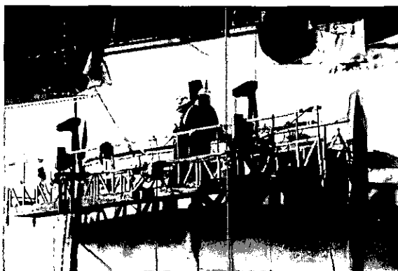
Fig. 11. The upper perimeter seal was installed just below the bottom of the concrete piers supporting the bridge deck
