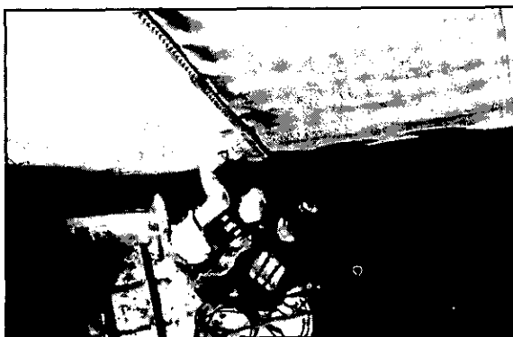
Fig. 10. External anchorage profile, with diver preparing to transit to underwater work. External dry profiles were covered by heat-welded PVC cover strips to prevent seepage along the set screw/hex coupler assembly. External underwater profiles were watertight connected to the internal ones
