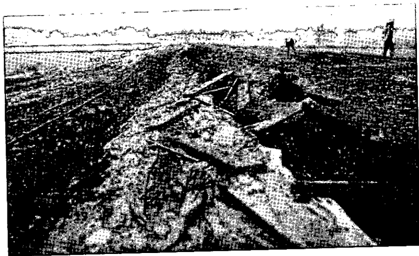
Plate 2 View of displaced puddle core on 20 July 1937
