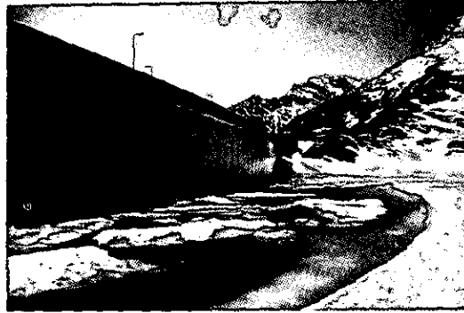
Fig. 11. Camposecco, a masonry dam, altitude 2337 m, where ice blocks driven by winds impact on the exposed PVC membrane installed in 1993
