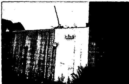
Fig. 9. Installation of the exposed membrane system at Nacaome dam.
