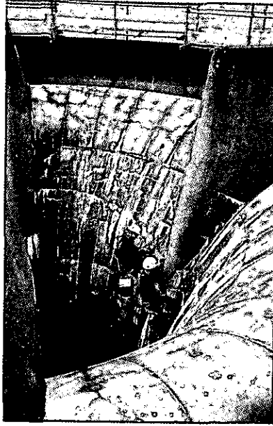
UPV testing on the flow splitter piers
