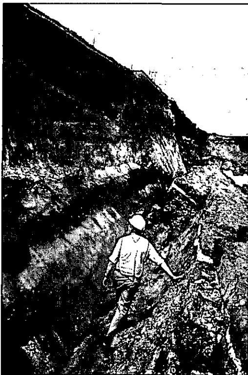
Figure 3. Failure of Carsington dam.
