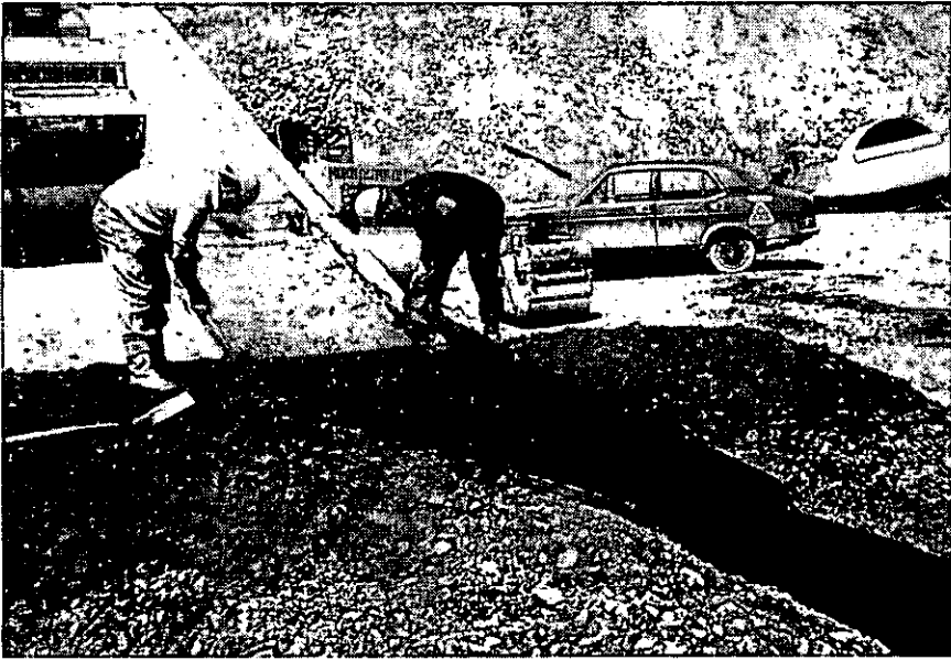
Figure 15. Base of bituminous core on roof of inspection gallery at Queen's Valley dam, Jersey.
