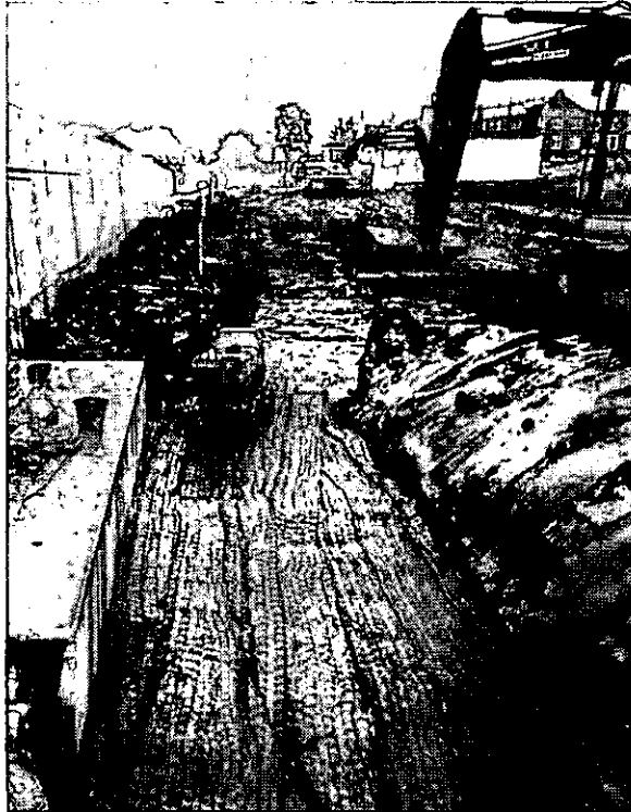
Figure 16. Trial compaction of clay fill against concrete structure in modification of Audenshaw reservoir.
