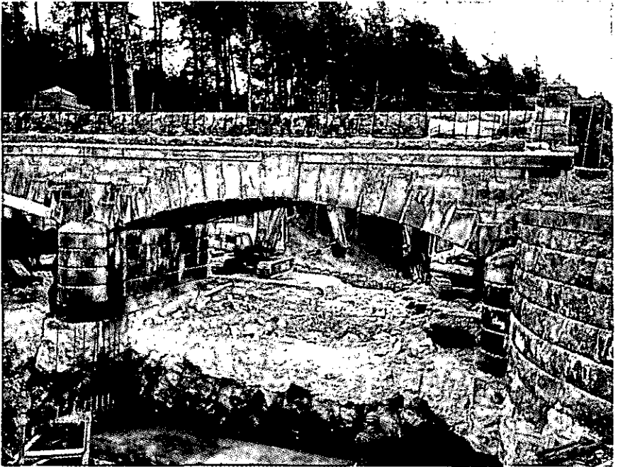
FIG 2. SPILLWAY BRIDGE EXCAVATION
