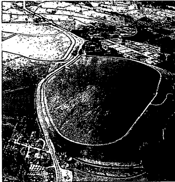
Fig 1. Aerial view of the Barrow Reservoirs
