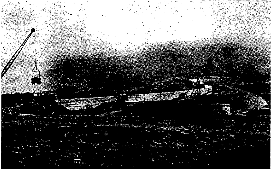
Fig. 5 — Dam during Construction (from Farrington, 1921)
