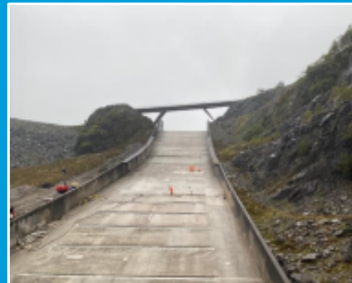
Llyn Brianne Spillway Maintenance
