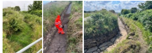
Spillway de-vegetation and masonry repair works in progress
