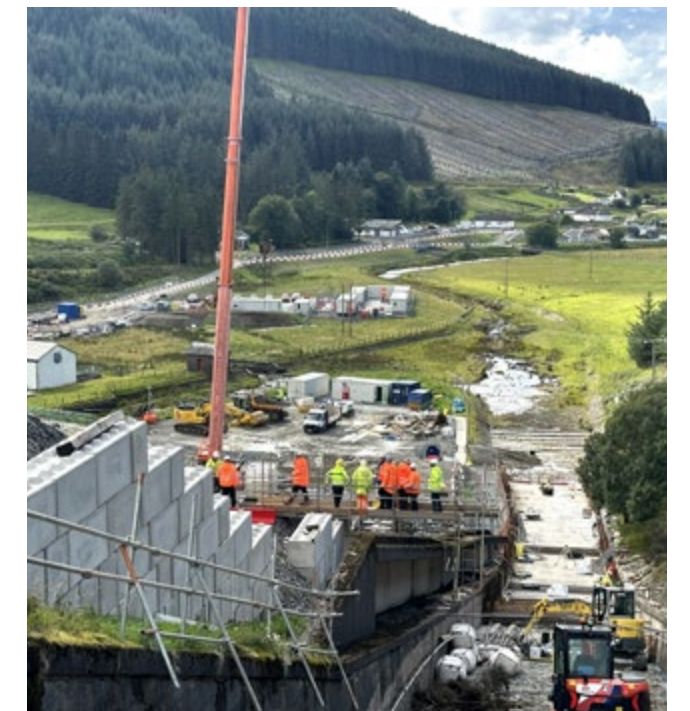
↑ View of the spillway chute under reconstruction
