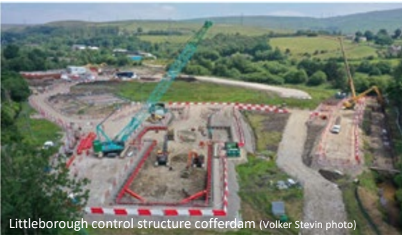
Littleborough control structure cofferdam (Volker Stevin photo)
