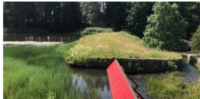
↑ Fish screen on a spillway crest - Jeremy Benn
