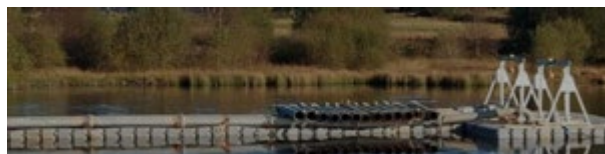
Temporary overpumping arrangements with large capacity pumps suspended from gantries on modular pontoon system with accessways for inspection and maintenance during the construction.
