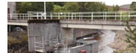
Works to install a compensation flow facility at the River Garry Intake
