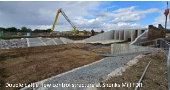
Double baffle flow control structure at Shonks Mill FDR
