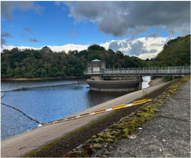
↗ Bellmouth spillway and valve tower along crest
