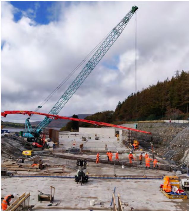
↑ New spillway at Llyn Celyn
