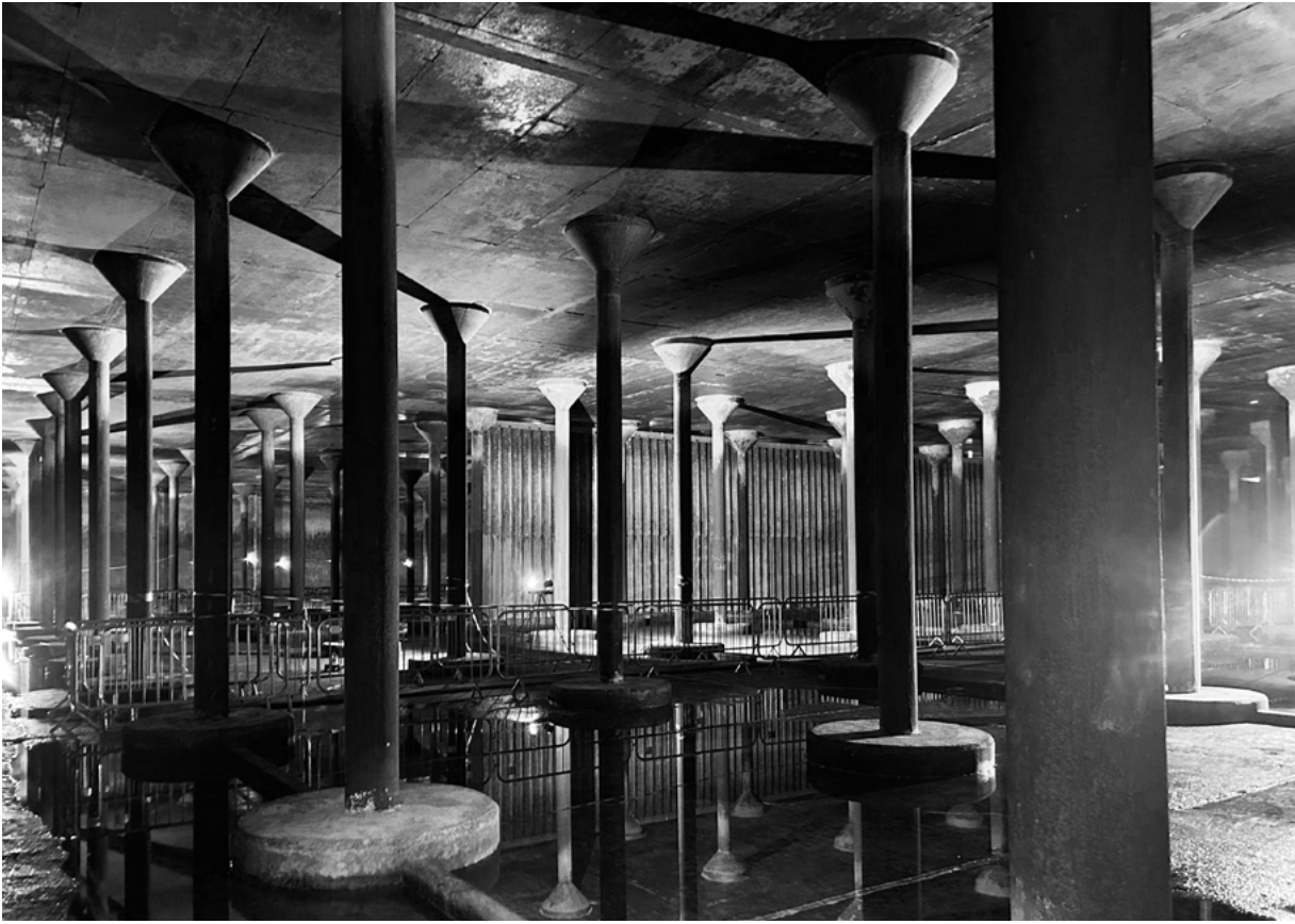
Phoebe Erskine Glenhove No 1 Service Reservoir, Cumbernauld, Scotland
