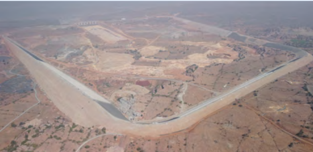
↑ Aerial view of upper reservoir, with upper power intake in distance
