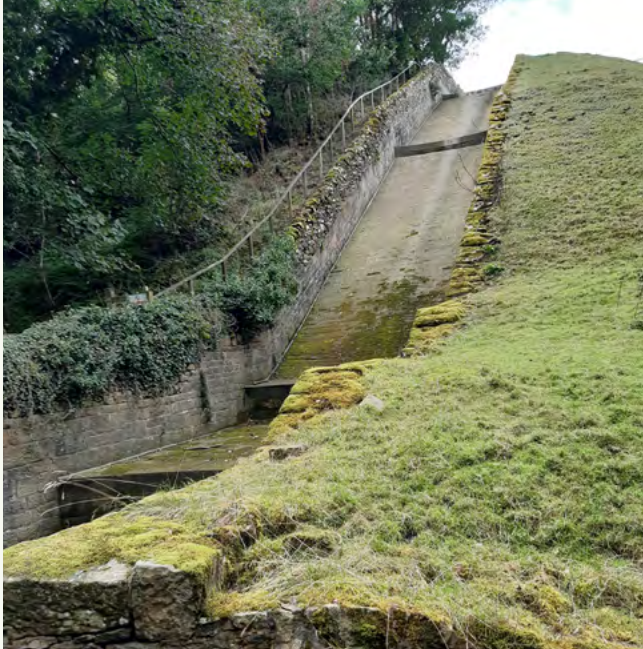
↗ Steep Ridgeway Primary Spillway
