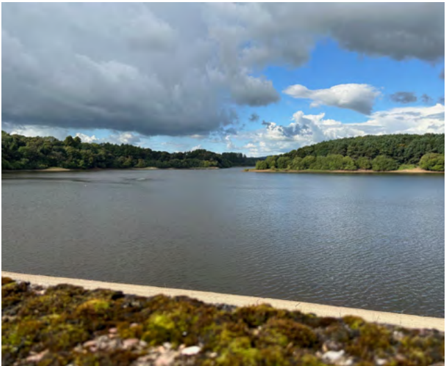
↗ View upstream from dam crest
