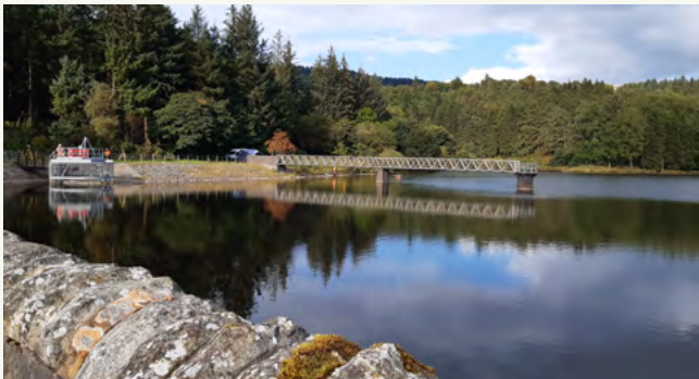
↘ Trentabank reservoir, view towards spillway and draw-off tower
