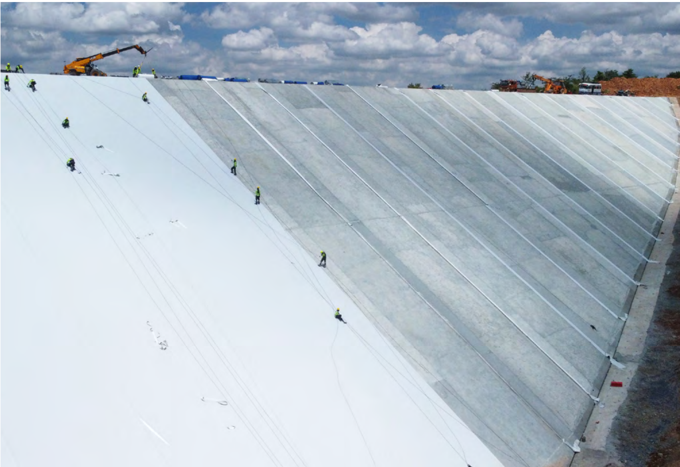
↑ Placing Carpi membrane on upstream face of lower dam
