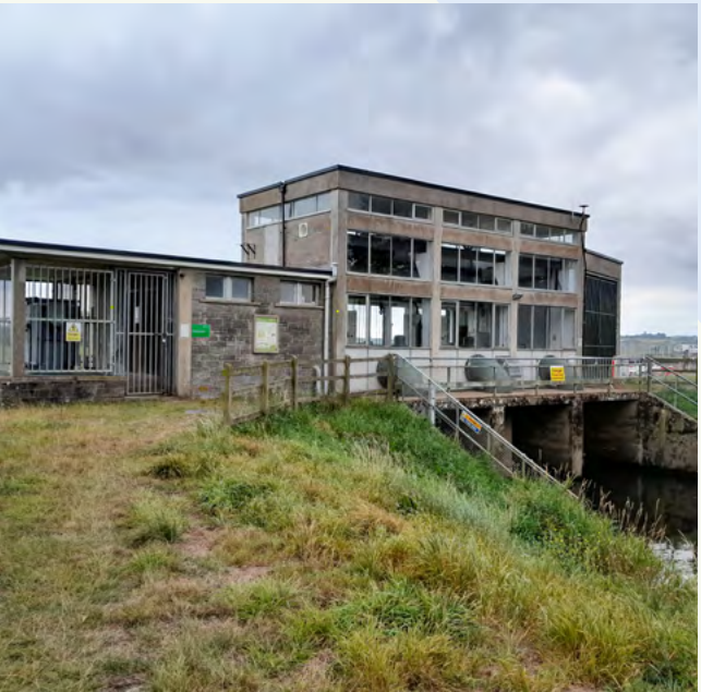
Middelney Pumping Station – Environment Agency
