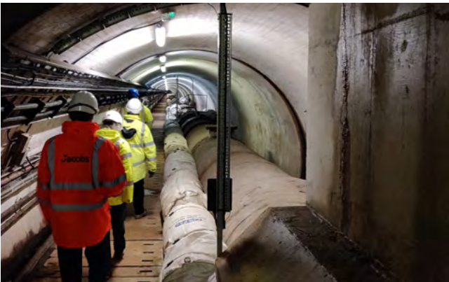
↑ Walking along the tunnel below Llyn Celyn
