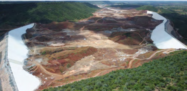
↑ Aerial view of lower reservoir
