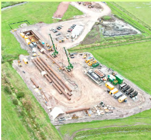
West Moor - Siphon replacement via direct pipe drilling
