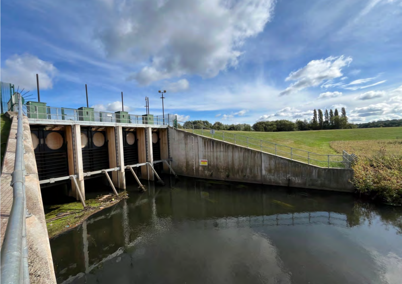
↑ Control structure with four 3m x 3m box culverts and penstocks
