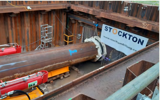
Tunnel boring machine – boring a new siphon under the river
