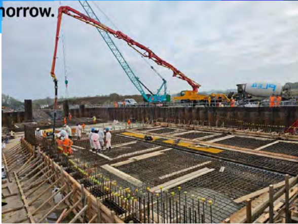
(Casting base slab of double baffle flow control structure at Shonks Mill Flood Detection reservoir)
