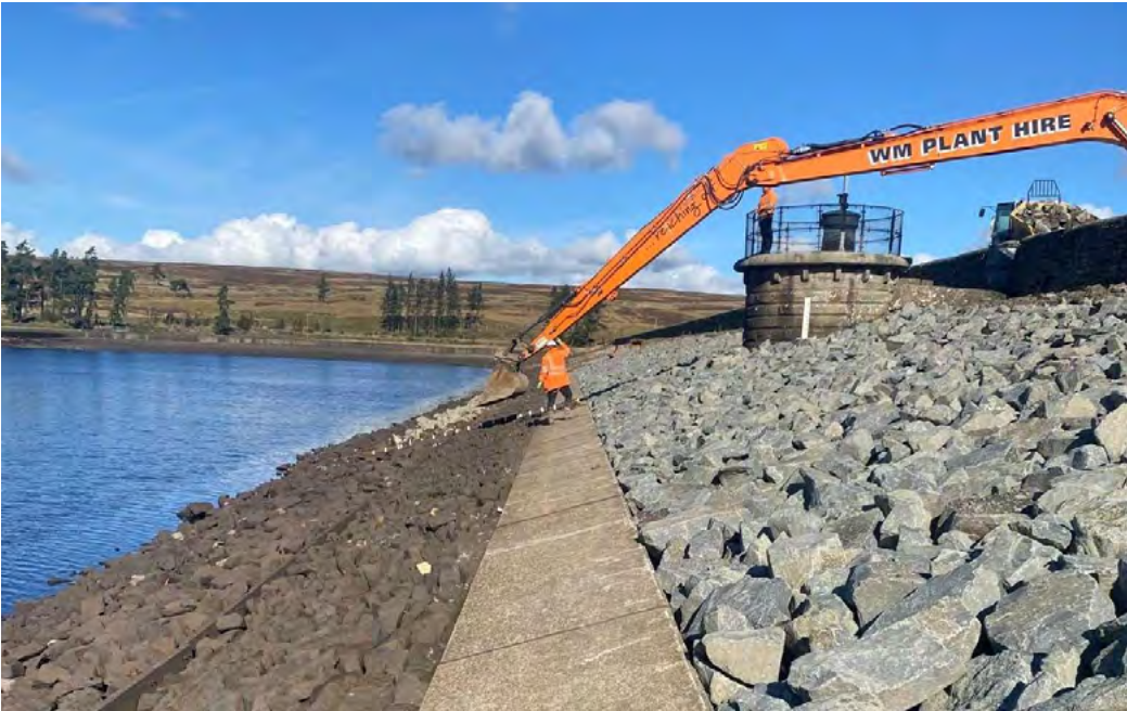
Waskerley Upstream Face Rock Works, 2024
