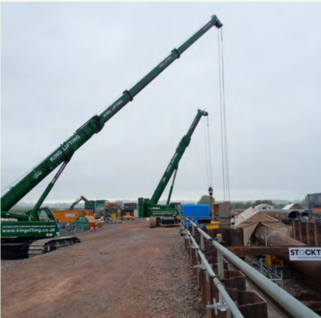
Specialist contractors Stockton Drilling progressing with boring new siphon under river channel
