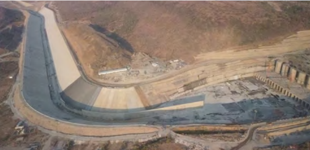
↑ Tailrace connecting channel with lower power intake on right
