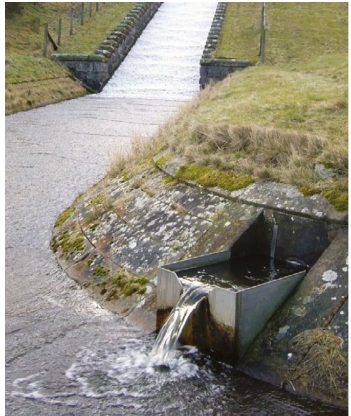
Vee-notch weir measuring toe drainage – Ian Hope
