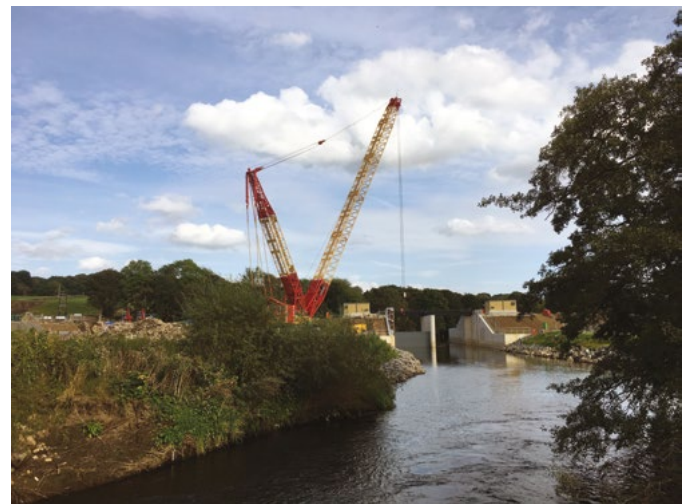
View of the flow control structure and 550tonne crane from upstream
