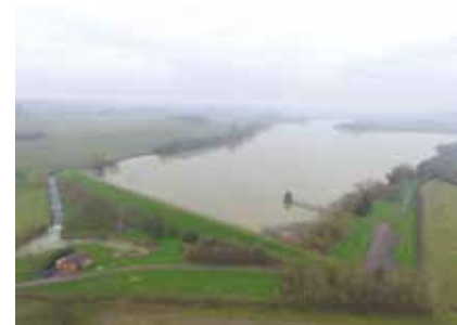
Stanford Reservoir was also built with a bywash channel which feeds into the spillway, allowing flow to be diverted around the reservoir.
