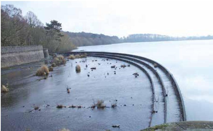
Young trees on a spillway requiring removal
