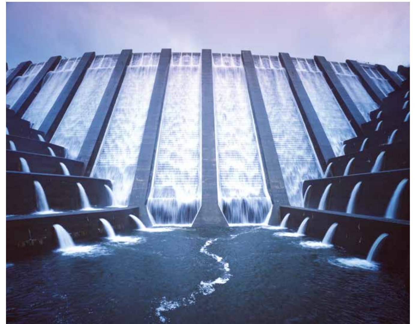
The spillways in operation at Clywedog safely passing flood flows after a rainfall event
