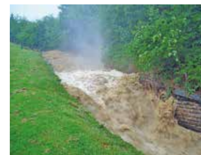
Boltby Reservoir, Yorkshire, in 2005 during and immediately after a major storm event. The masonry spillway protecting the dam failed as illustrated.
