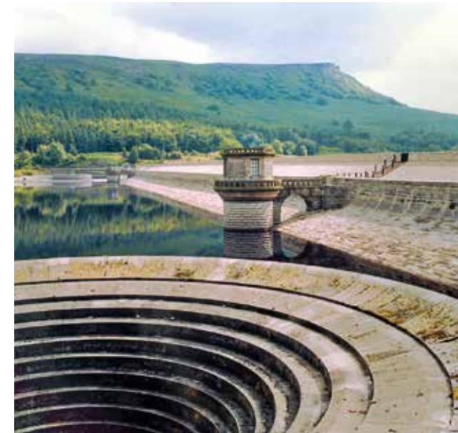
The drop shaft spillway at Ladybower Reservoir is pictured; both dry and spilling
