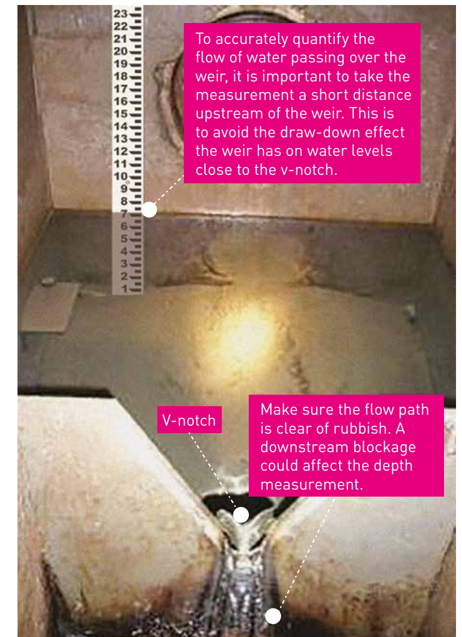
V-notch weirs are found at the end of toe drains.
