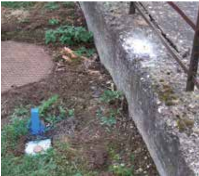
Examples of monitoring pins
