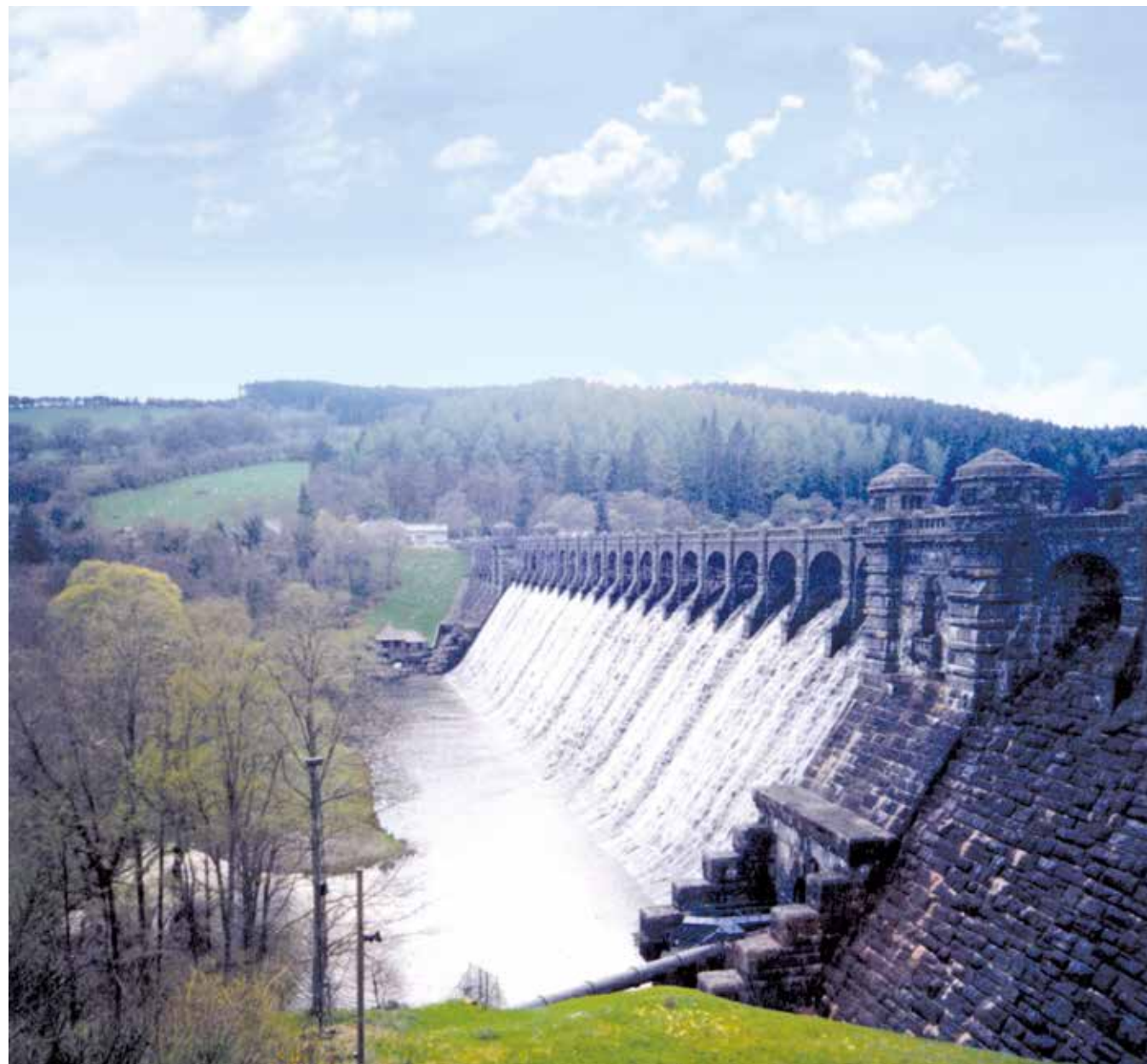
Excess water safely flowing over the spillway at Lake Vyrnwy - a typical gravity dam
