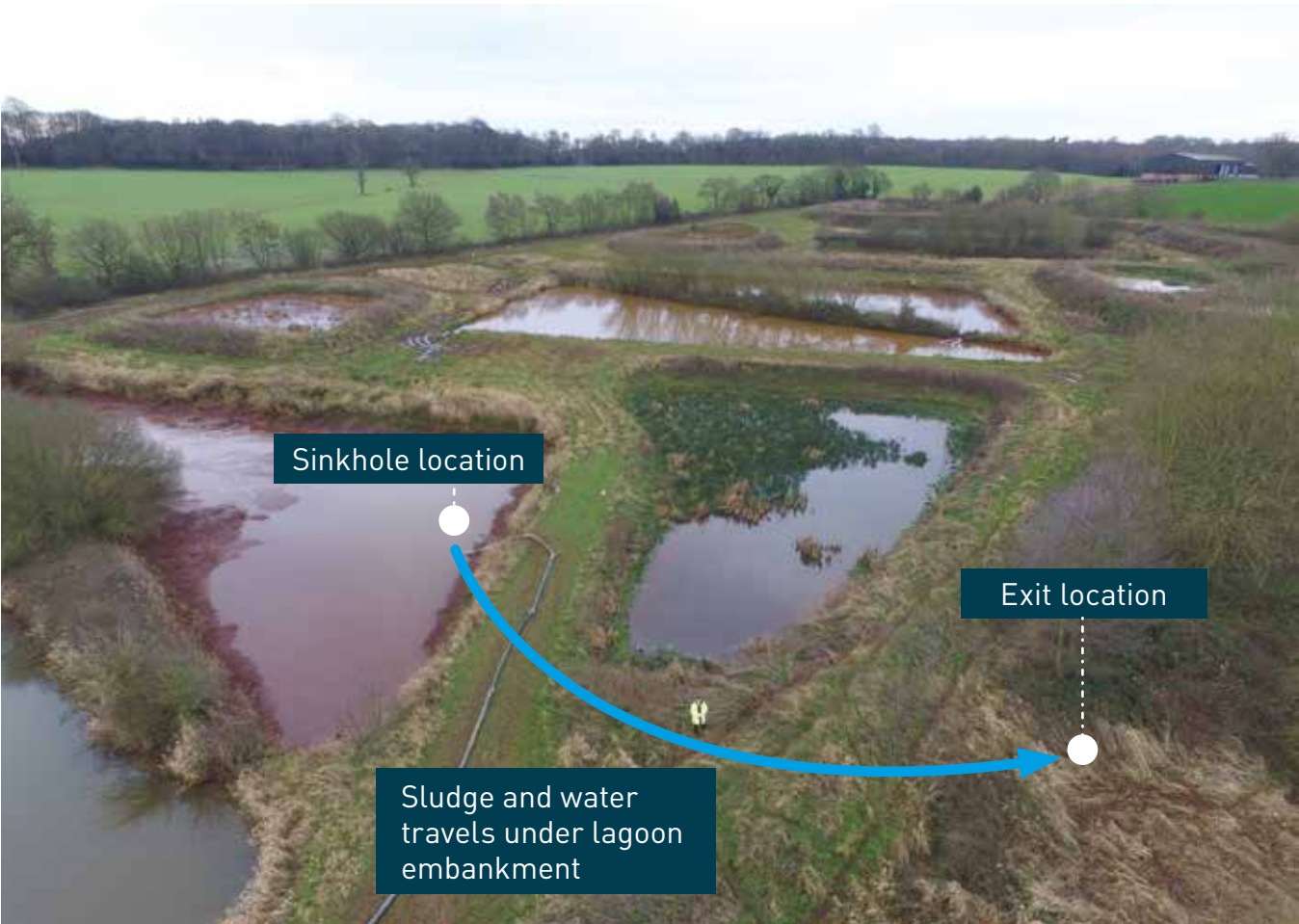
A mixture of sludge and water escaped from a lagoon at Melbourne WTW due to foundation failure of one of the embankments. The likely cause was water penetrating through the foundation of the non-engineered lagoon embankment.
