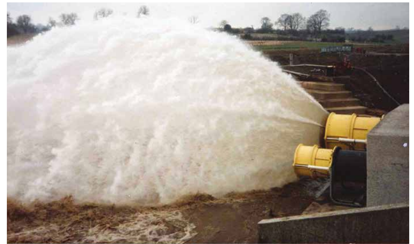
Exercising the scour valve at Carsington Reservoir
