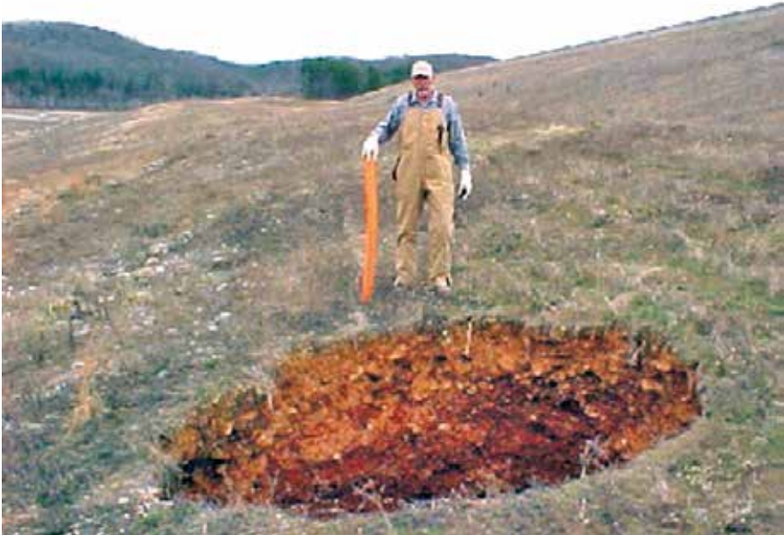
Sink hole formed following hidden internal erosion
