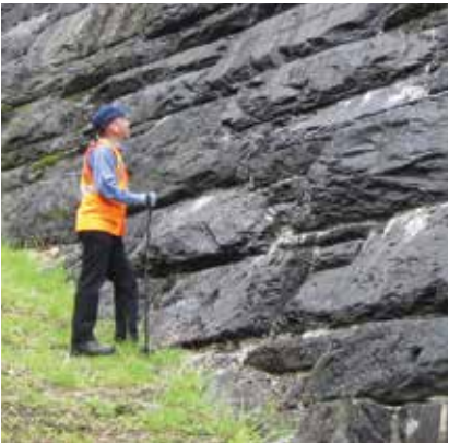
Looking for signs of movement in the stonework at Lake Vyrnwy.
