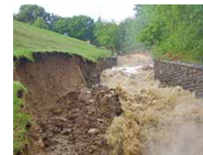
Boltby Reservoir, Yorkshire, in 2005 during and immediately after a major storm event. The masonry spillway protecting the dam failed as illustrated.
