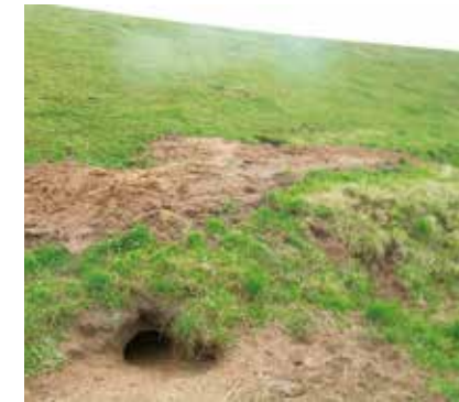
Entrance to badger sett on earth embankment dam
