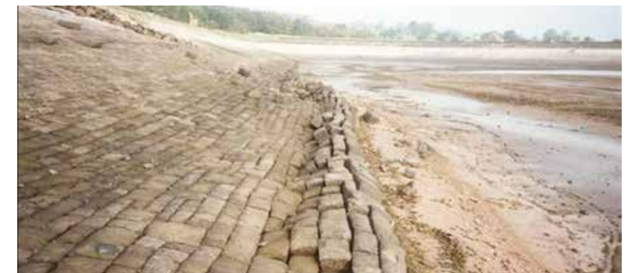
An irregular waterline shows a slip on the upstream face, with a bulge at the toe and distortion of the pitching revealed when the water level is dropped
