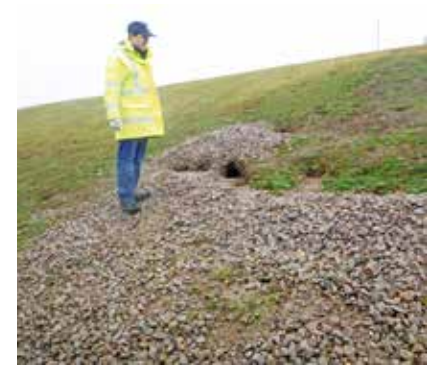
Example of rabbit activity on the downstream face of Draycote Reservoir
