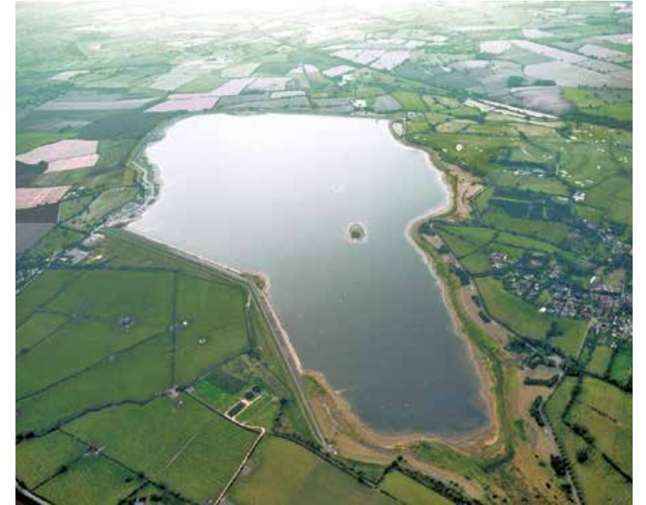
Draycote is a non-impounding reservoir made up from 6 embankment dams.
