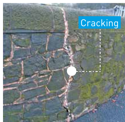
Bartley Reservoir - wave wall
