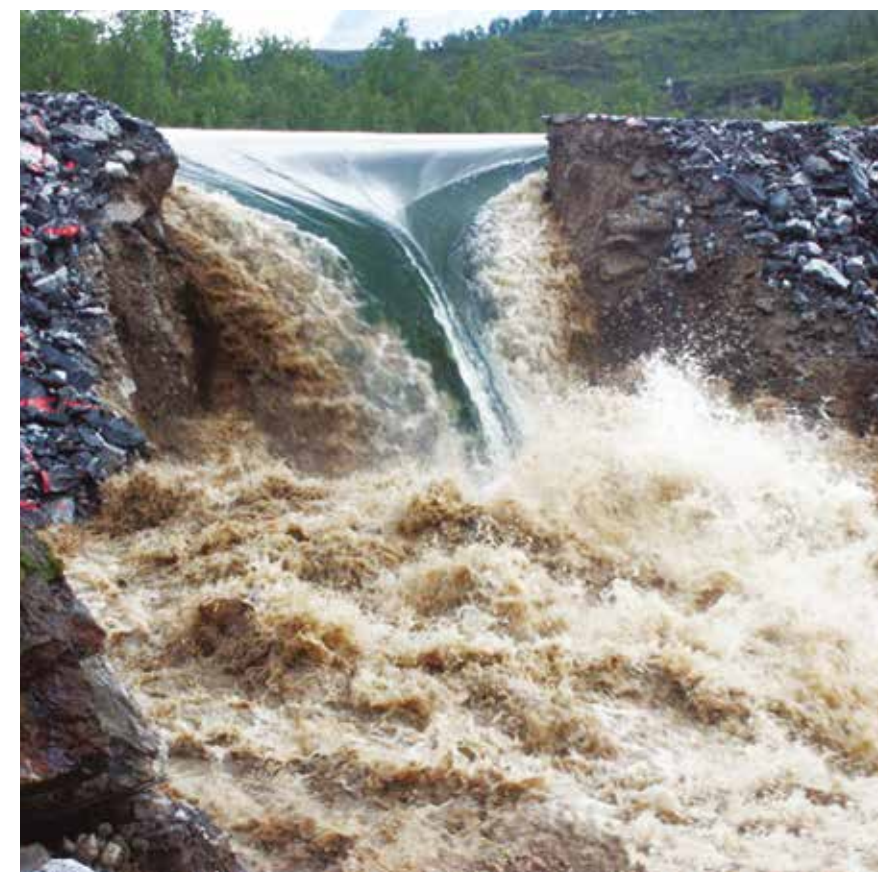
Water released from the reservoir by a breach in the dam causes further erosion.
