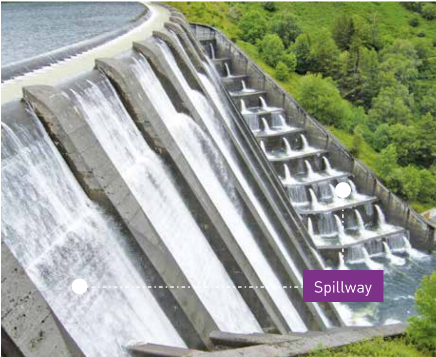
Overtopping of Clywedog Dam showing two types of spillway in use.
