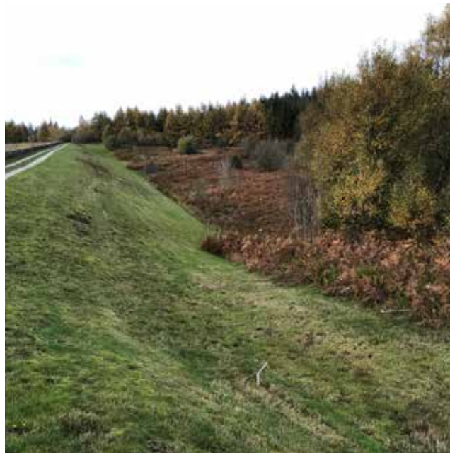
Progressive overgrowth along the toe of Pendinas Reservoir
