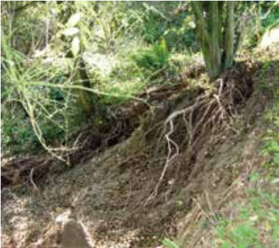
Localised erosion around tree trunk following overtopping event.
