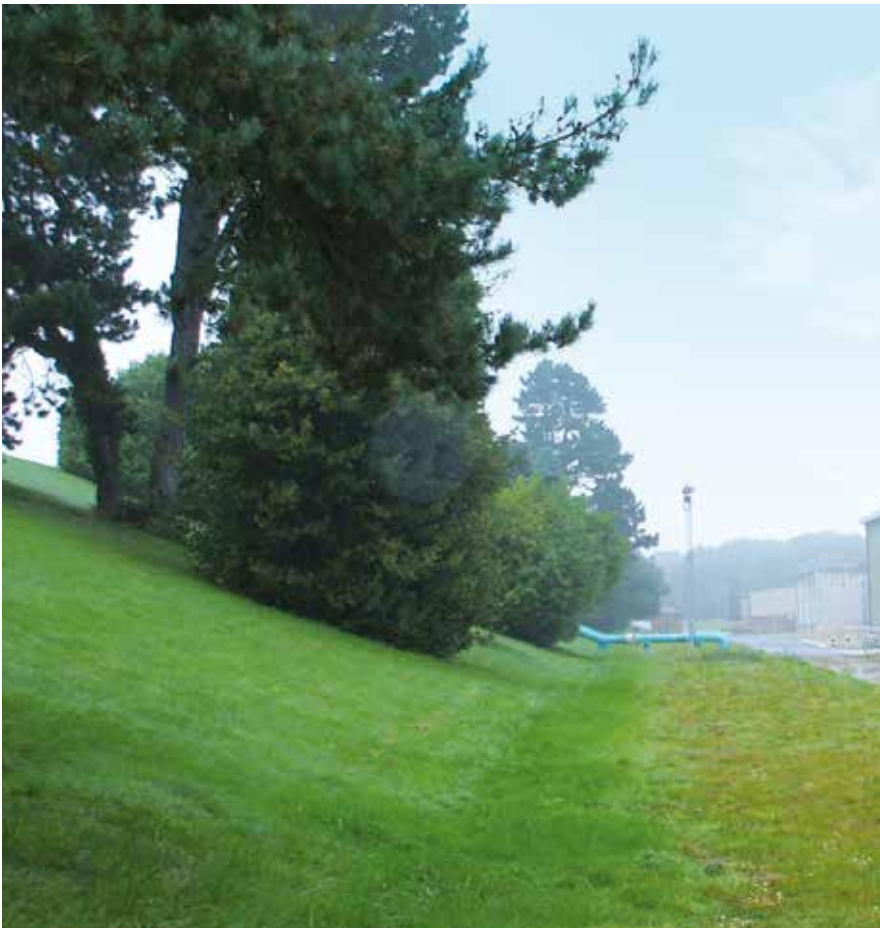
Trees growing on an embankment dam, which is far from ideal.
