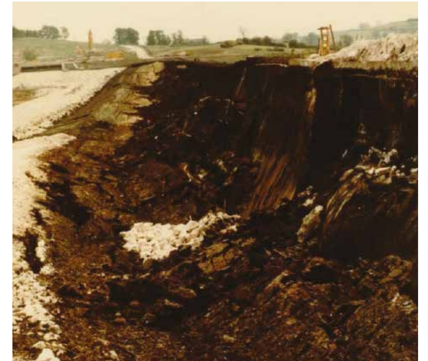
The dam after the slip failure
