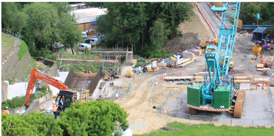
Figure 4 View of the construction site June 2026.
