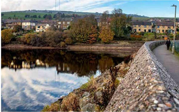
Figure 1 Slaithwaite Reservoir looking north.
