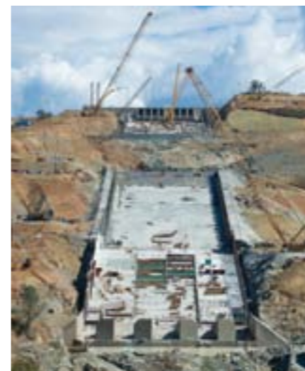
Photo of the primary spillway at Oroville Dam on September 22, 2017, under construction as part of the recovery project in response to the February 2017 incidents (photo courtesy of California Department of Water Resources).
