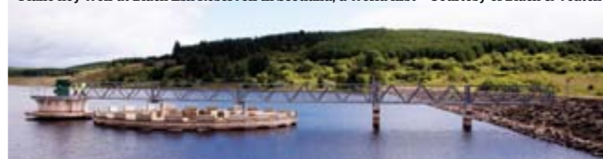
Piano key weir at Black Esk Reservoir in Scotland, a world first – Courtesy of Black & Veatch
