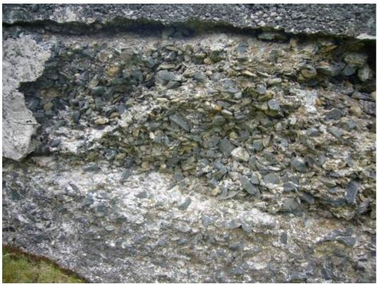
Figure 5-25 Typical poor concrete of Eigiau dam showing honeycombing and lack of fines
