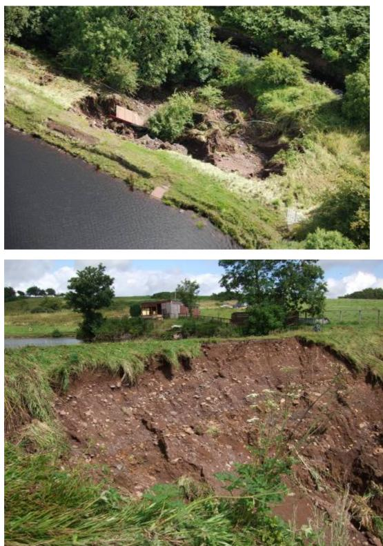
Figure 5-20 Erosion of the downstream shoulder fill due to overtopping at Maich Water
