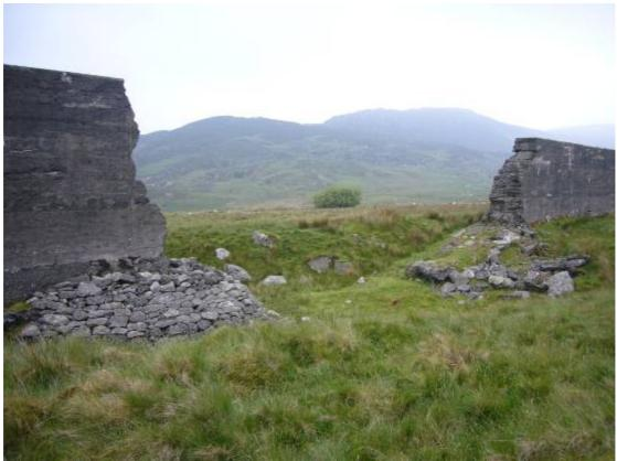
Figure 5-24 The breach at Eigiau dam (taken 2009)
