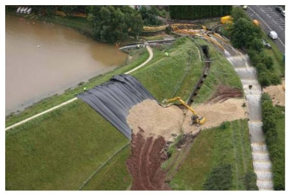
Figure 5-19 Temporary remedial works to stabilise the embankment following the incident at Ulley dam
