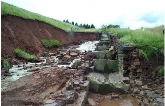
Figure 5-18 View of collapsed stepped masonry spillway and adjacent erosion of embankment fill at Ulley dam
