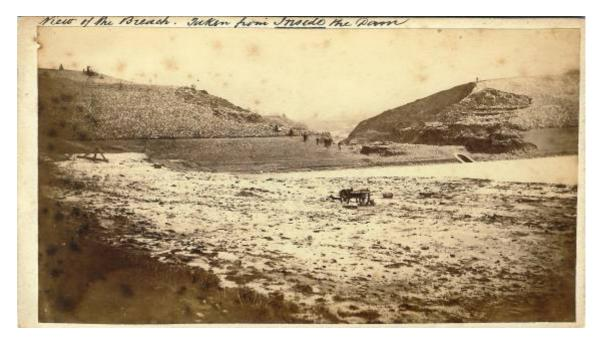
Figure 2-3 Postcard photograph of the Dale Dyke dam breach (courtesy of C Hoskins)
