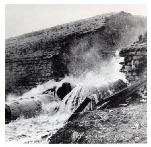
Figure 5-7 Breach of the embankment along the line of the recently constructed drawoff tunnel at Warmwithens (from *Engineering Now*, No.4, December 1970)
