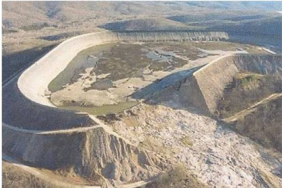
Figure 5-32 Breach through Taum Sauk embankment
