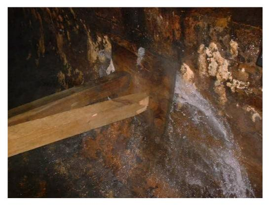
Figure 5-11 Leakage in the draw-off culvert at Yarrow embankment and temporary plug (after Gardiner *et al.*, 2004)
