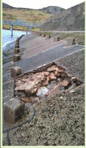
Photo 1: hole in concrete slab
