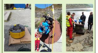
photo 3: from left, inflatable plug, plate and bellmouth.
