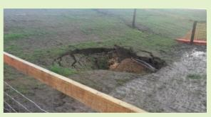
Photo 1: sinkhole at toe of embankment
