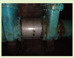
Photo 1: Short section of steel pipe on the scour pipe
