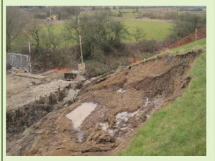
Photo 2: saturated fill material during excavation March 2016
