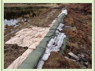
Photo 2: western breach location, following works to seal the breach
