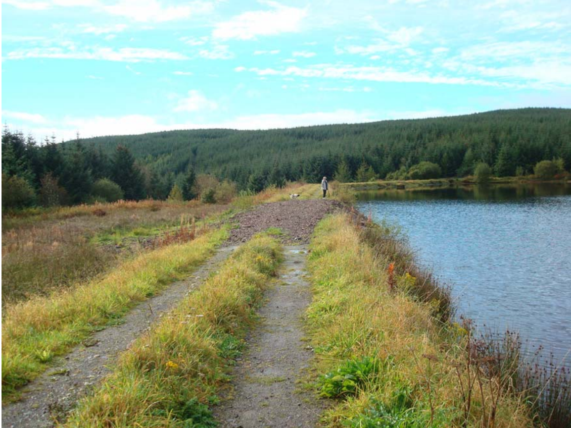
Photo 1: Reservoir affected by Incident 345
