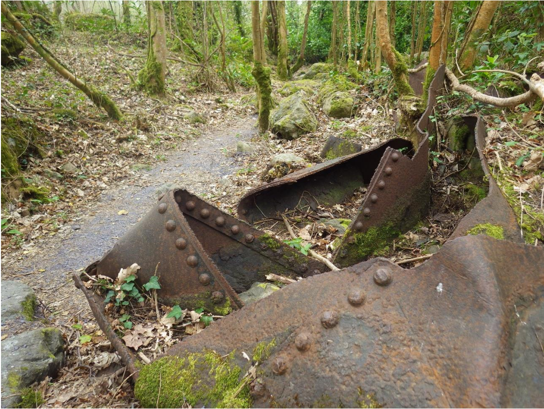
Figure 3. the water pipe which fed the Dolgarrog aluminium works lies crumpled amongst boulders and trees.
