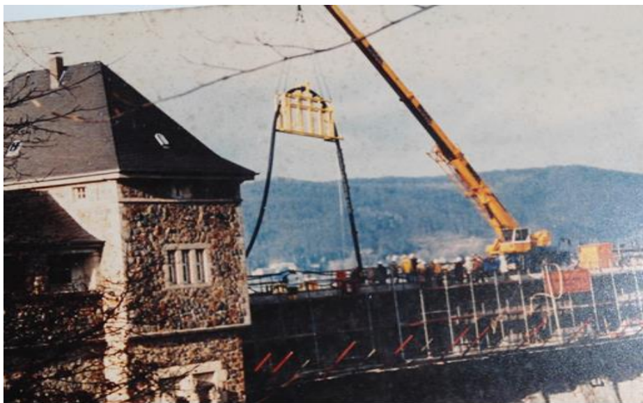
Old photograph: showing installation of anchors at Eder dam.
