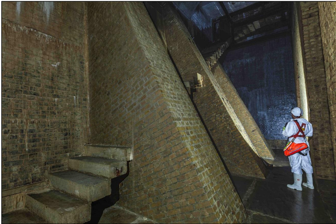
Maiden Lane Service Reservoir
