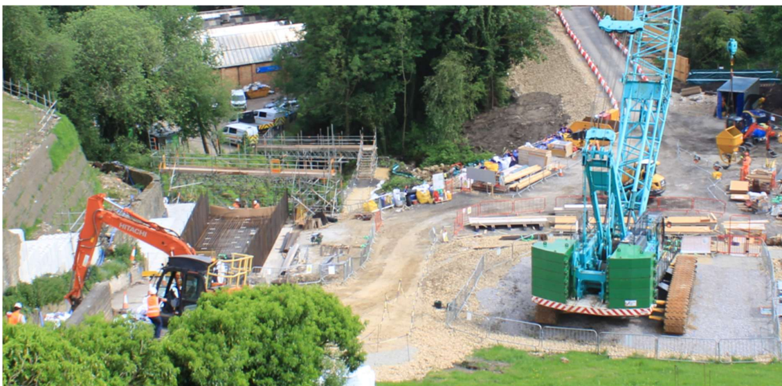
Figure 4 View of the construction site June 2026.
