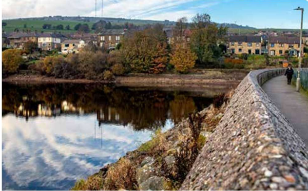
Figure 1 Slaithwaite Reservoir looking north.
