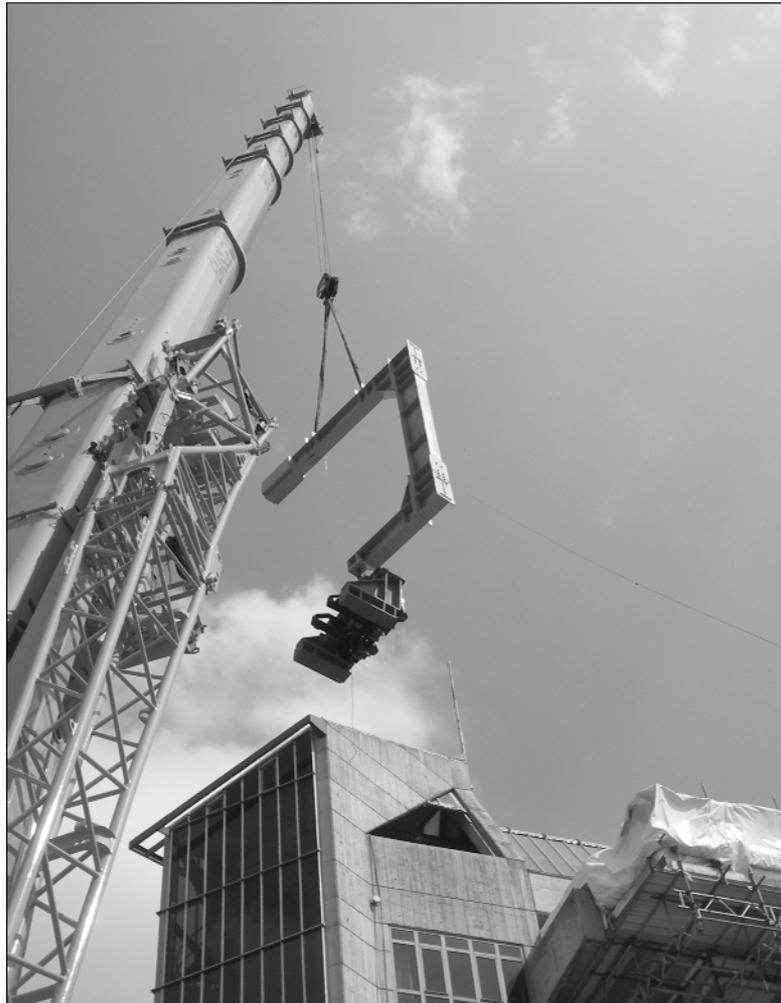
Figure 4 Lift operation using C hook
