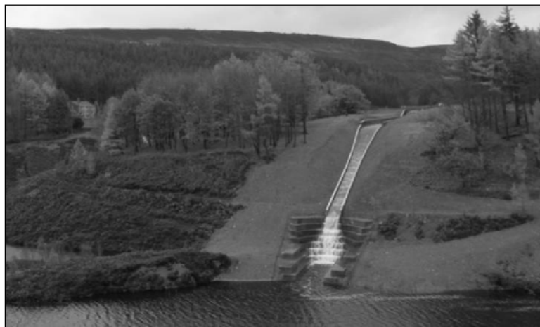
Figure 12. Completed works at Riding Wood
