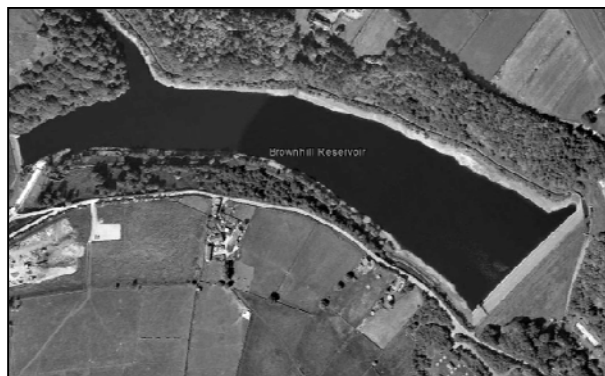
Figure 13. Aerial view of Brownhill reservoir
