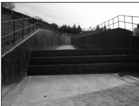
Figure 8. Ramsden crest bridge
