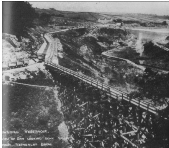
Figure 2. Rake Dike trestle bridge above Brownhill
