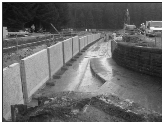
Figure 17 – Yateholme pre-cast concrete units being installed
