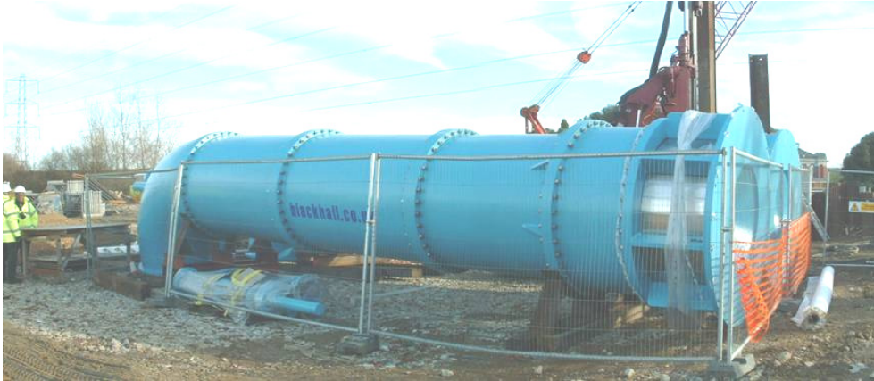
Figure 4: Submerged discharge valves awaiting installation.
