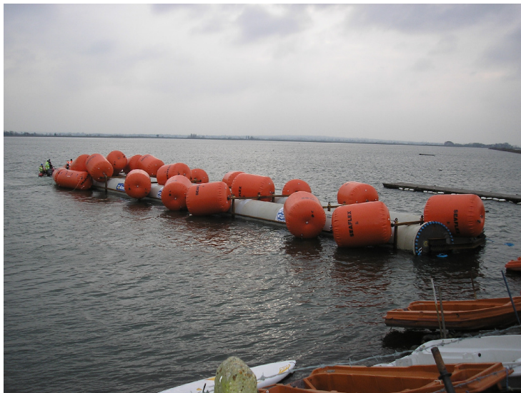
Figure 6: Pipework assembly being floated across Queen Mary Reservoir
