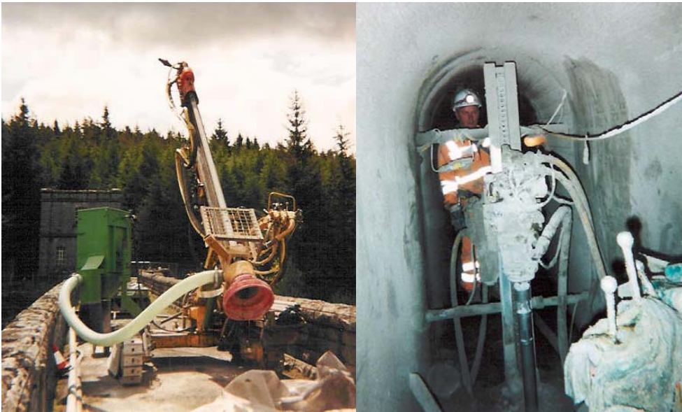
Figure 4 Drilling equipment at Laggan Dam crest and gallery
