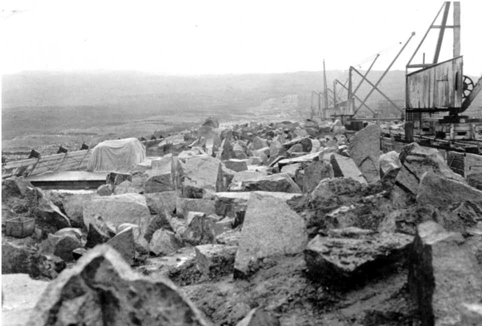
Figure 2 Displacer blocks on lift joints at Blackwater Dam
