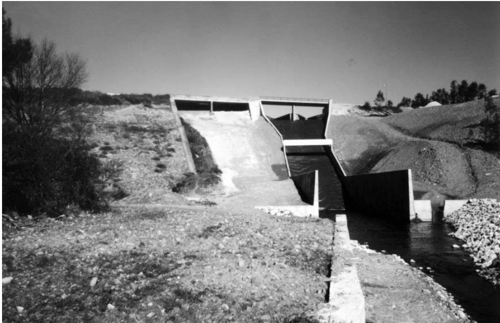
Figure 2. New spillway of the Pisco dam alongside the old one.
