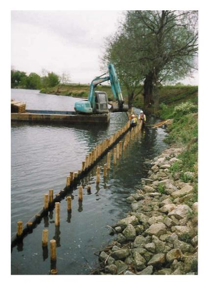
Fig. 5 View of revetment system being placed
