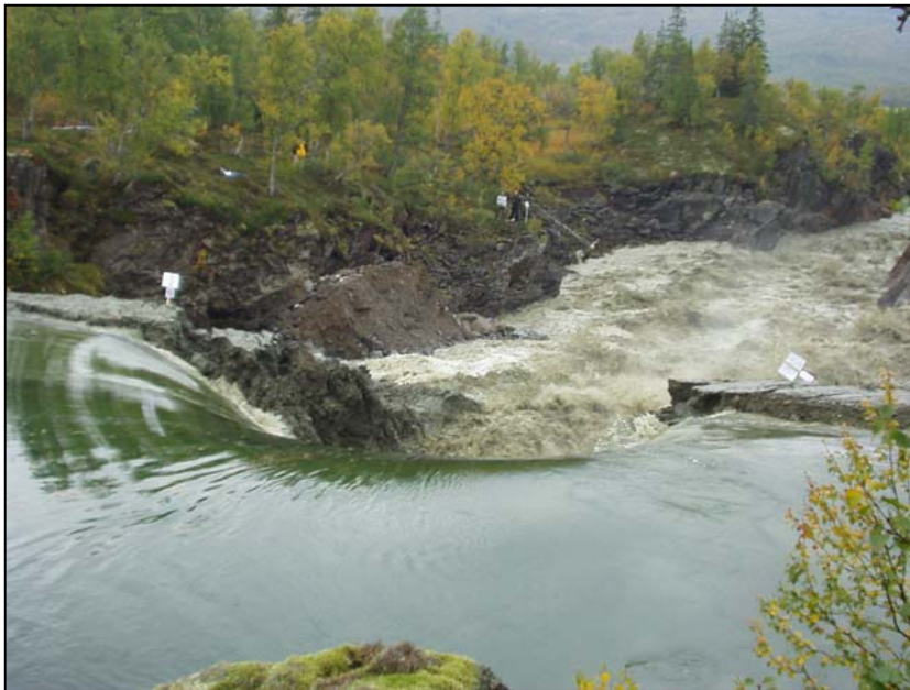
Plate 2: Weir control section
