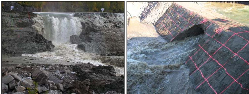
Plate 1 Field Test #1 (left) and Field Test #5 (right)
