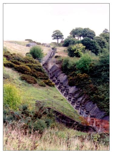
Plate 2: Eastern cascade channel on the left mitre of the embankment
