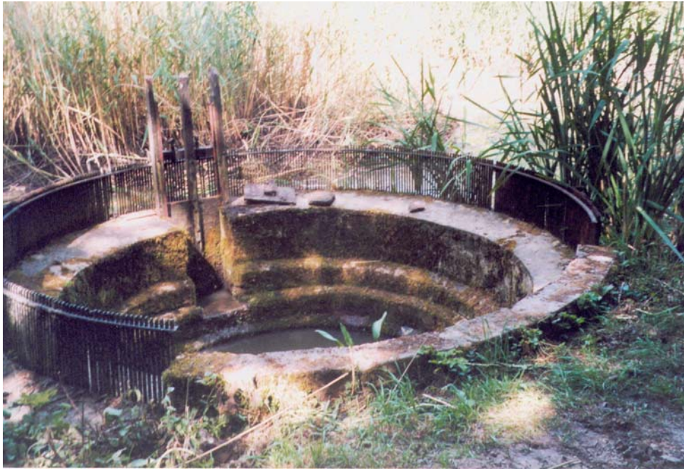
Figure 4. Glory Hole Spillway at Marston Pond prior to lowering by 450 mm.
