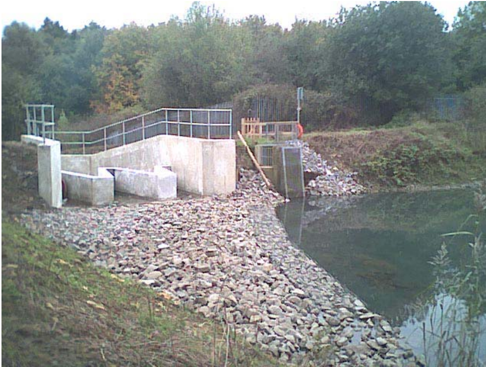
Figure 2. New Labyrinth Spillway at Weldon Lagoon
