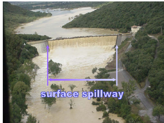
The flood mitigation dam of La Rouvière on the Crieulon Creek on September 9 th , 2002
