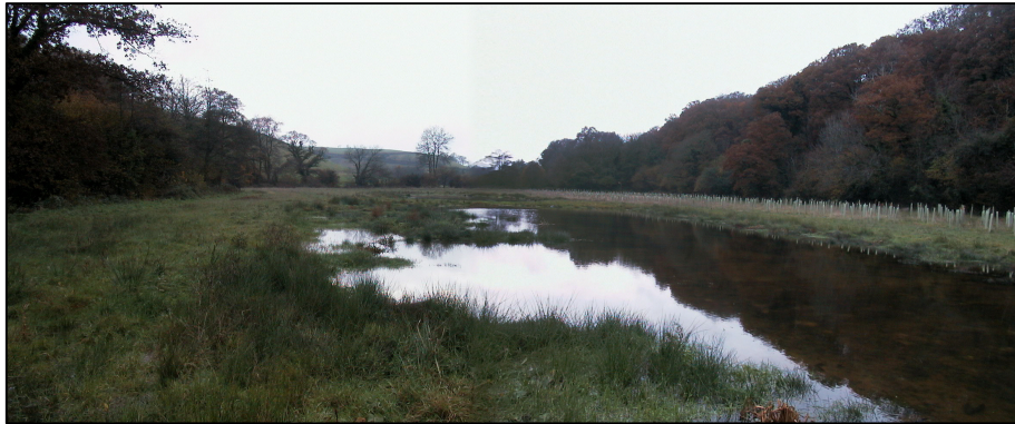
Figure 5: Photograph of washland area one year after construction
